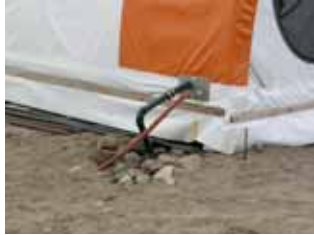
Greywater Drainage From Kitchen Module
