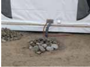
Greywater Drainage From Ablution Module
