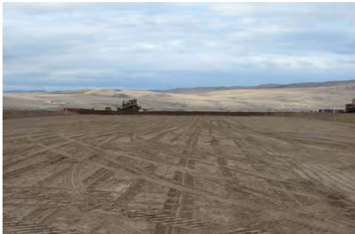
Photo 1: Shaping the bulk fuel storage area floor and berms.
