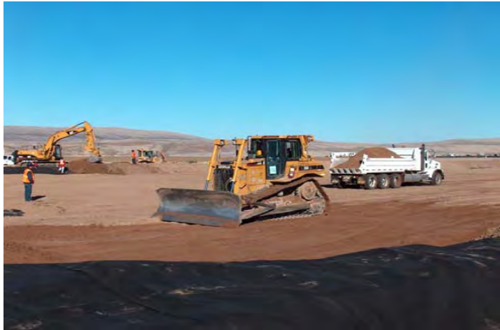
Photo 6: Placement of granular material overtop of non-woven geotextile.
