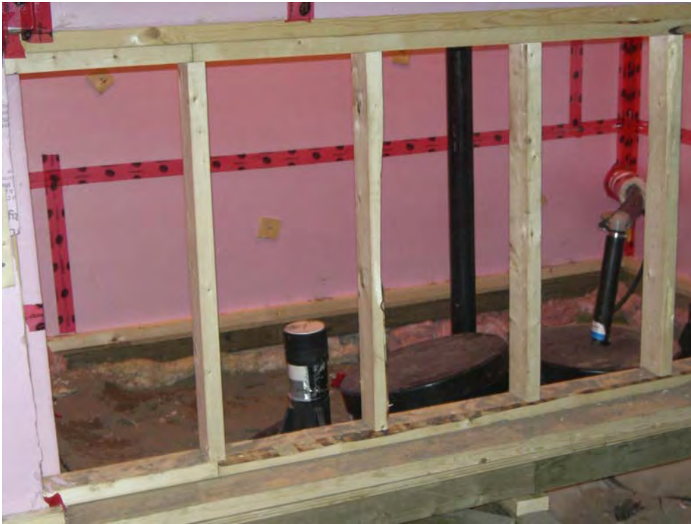
Photo 5: Final pumping chamber going to the PWSP
