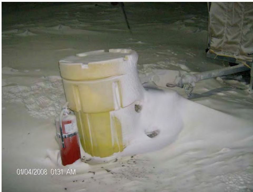
Spill kit at aviation fuel dispenser.
