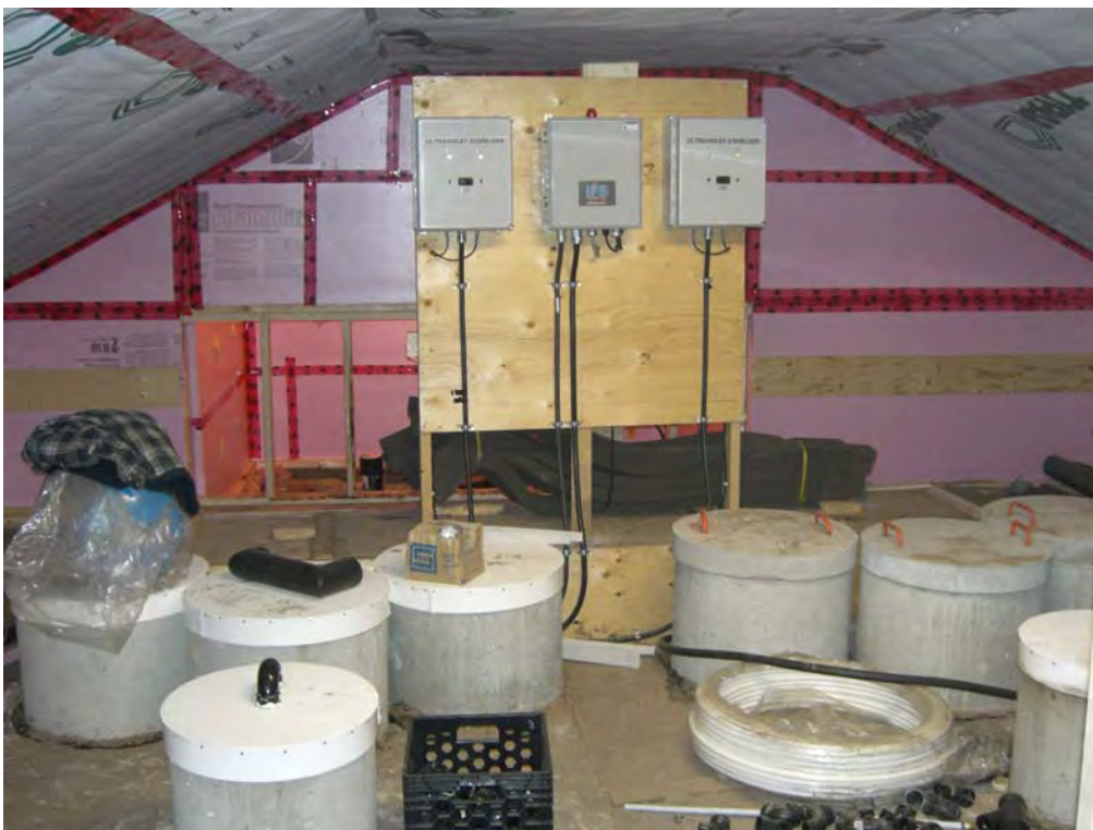
Photo 4: Aeration, final process and UV tanks
