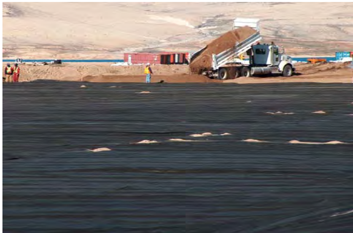
Photo 5: Upper layer of non-woven geotextile in place.
