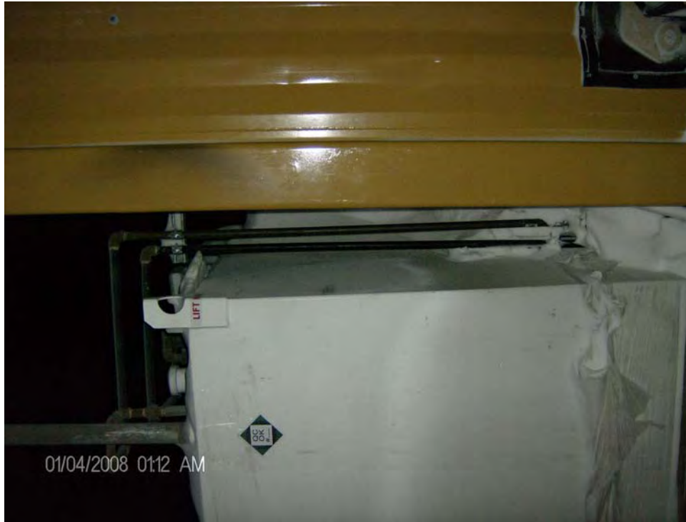
Milne: Double-wall fuel tank for stand-by generator
