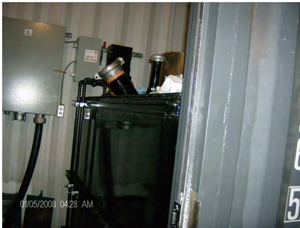
Mary River: Double-wall tank for main generator
