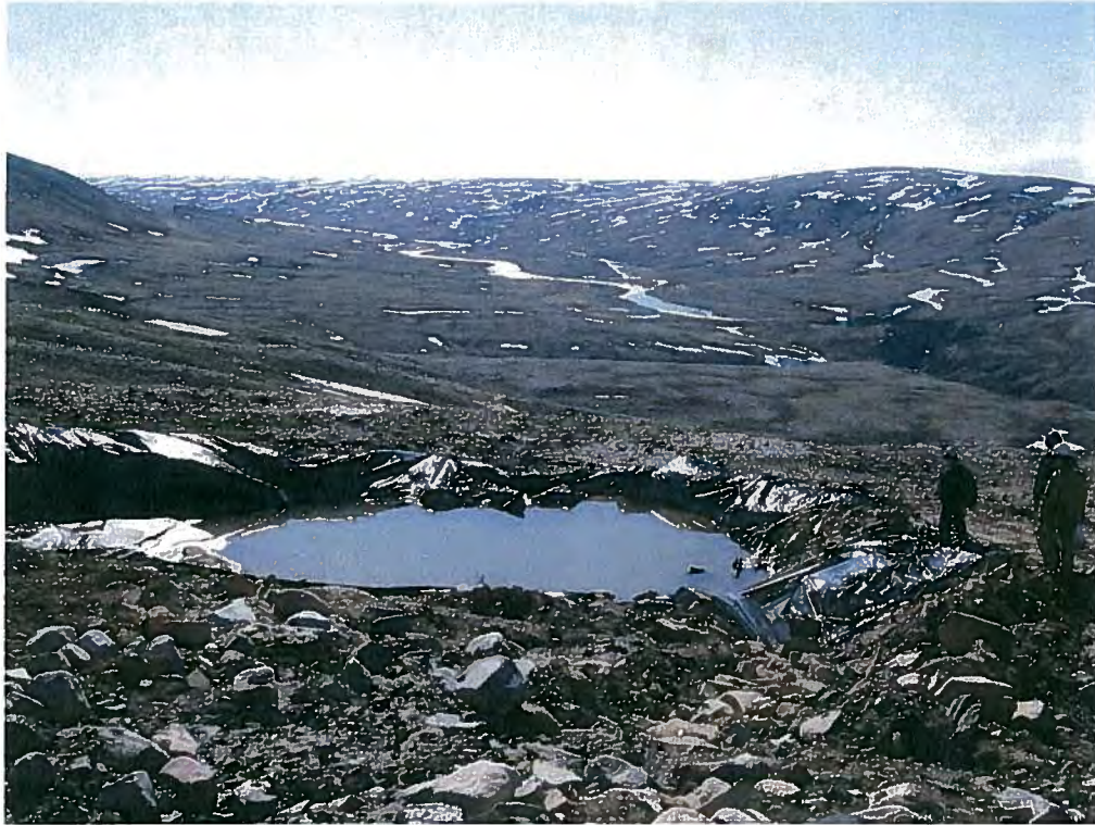
Photo 11: Axial sump (SU 6) with liner (photo 1)
