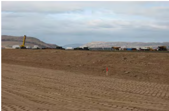
Photo 2: Floor and berm prior to liner placement.
