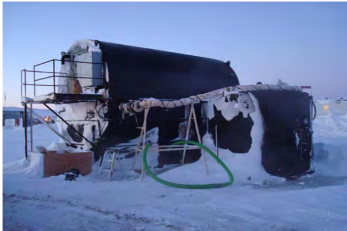
Photo 61: Wastewater Treatment Facility (rotating biological contactor) installed at Milne Inlet in 2007.
