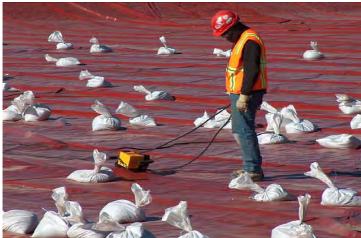
Photo 4: Welding of liner seams.
