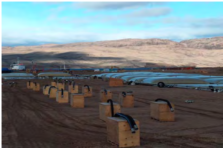
Photo 4: Fuel bladders and pumping systems in place.
