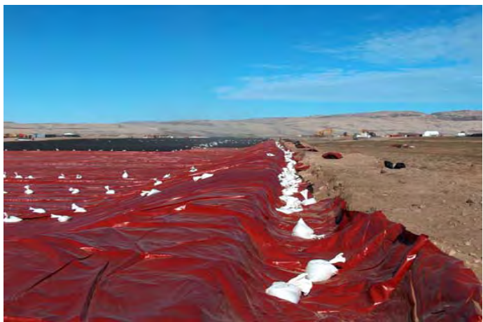
Photo 3: Liner placement, including anchor trench.
