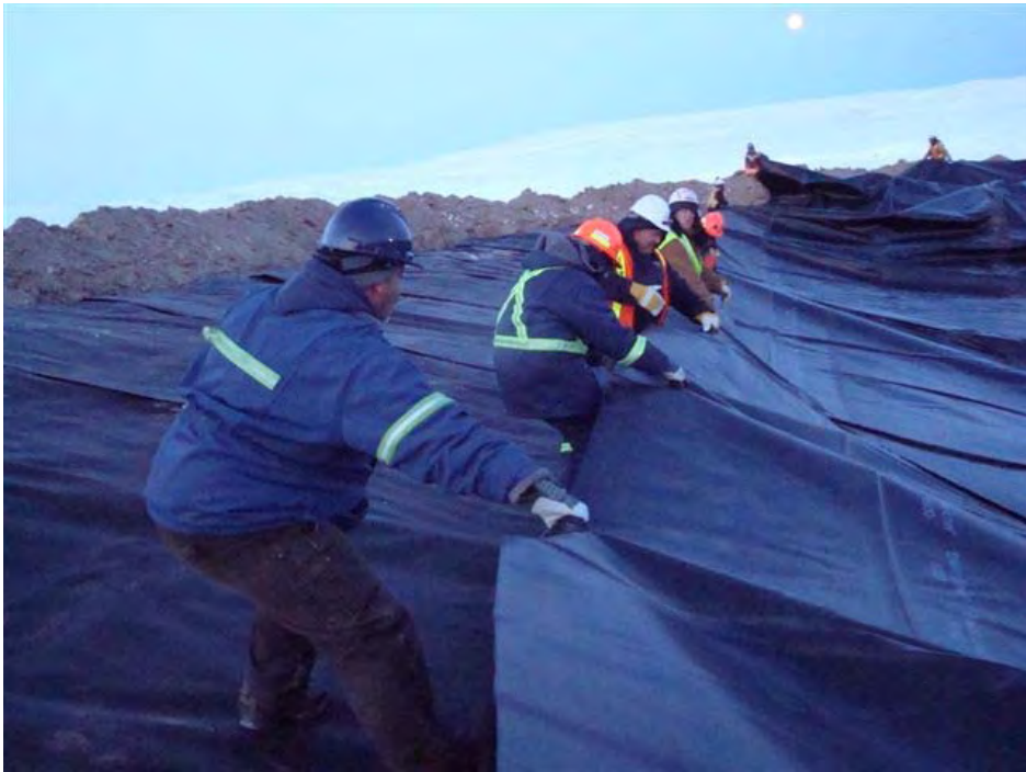
Photo 2: Crew is installing the liner at PWSP #3
