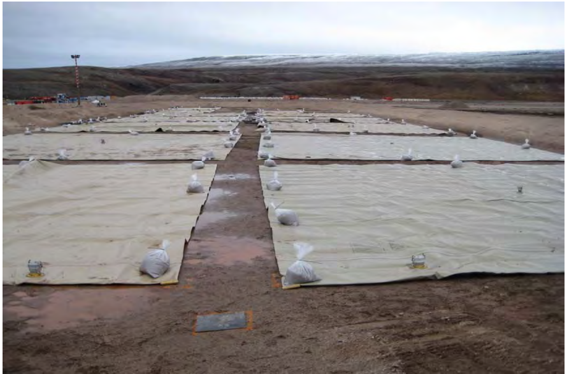
Mary River Fuel Containment Facility (during bladder installation)
