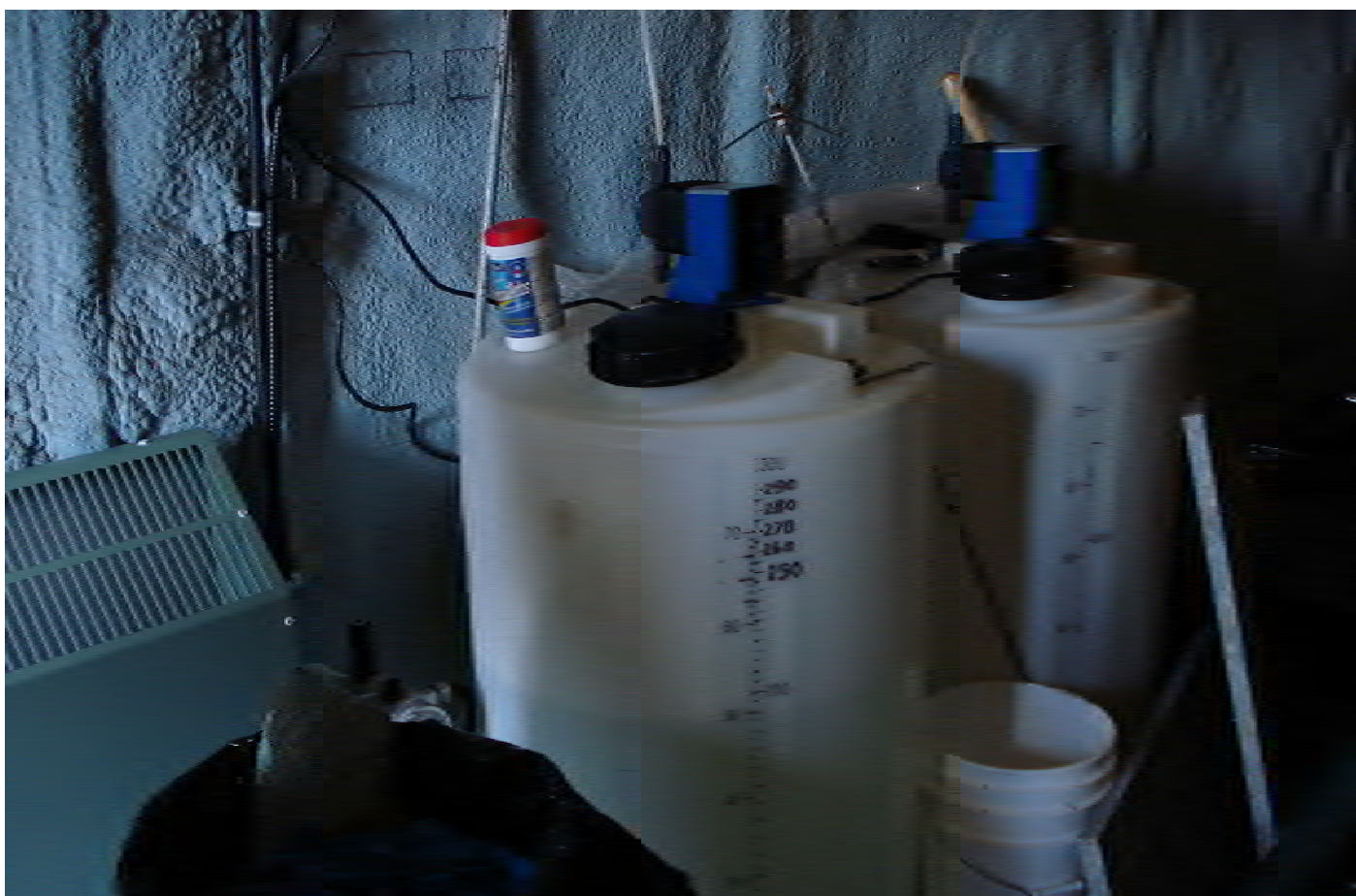
Photo 4: Alum & Sodium Bicarbonate Tanks
