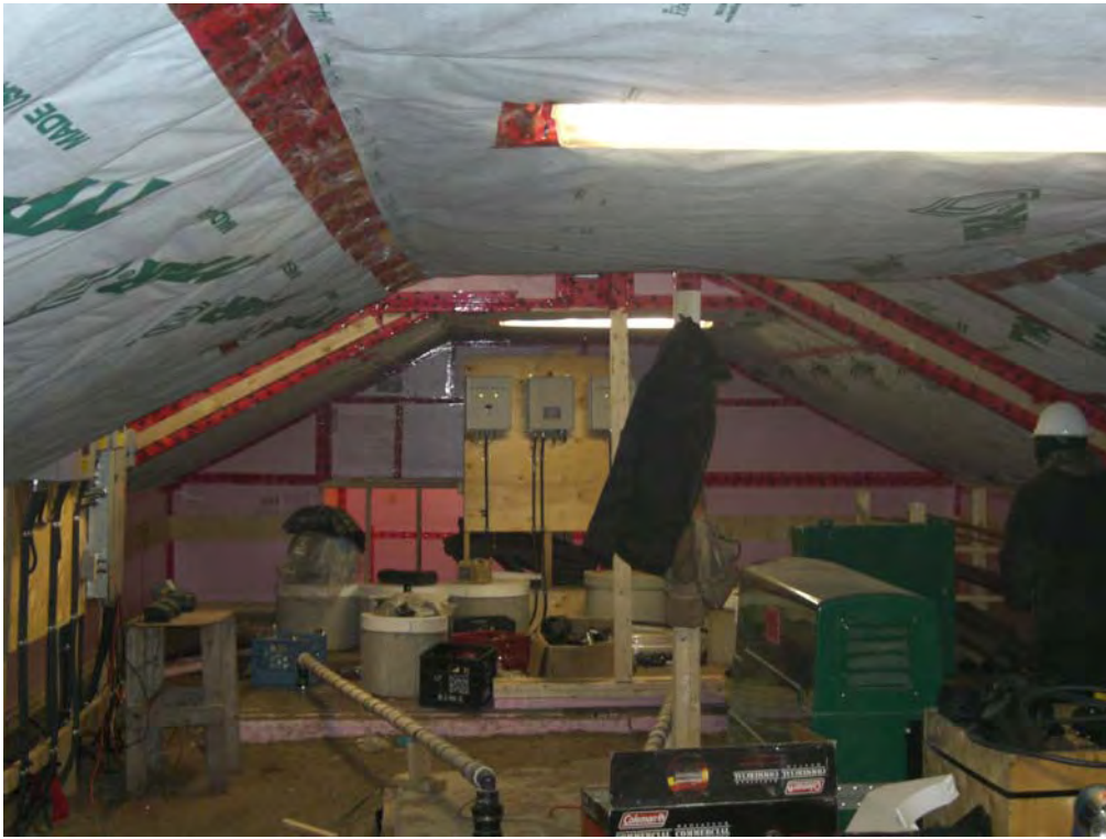
Photo 3: Pre-treatment tanks and aeration chamber at the bottom of the photo
