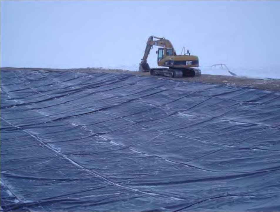
Photo 5: The top of berm is being covered with granular material.
