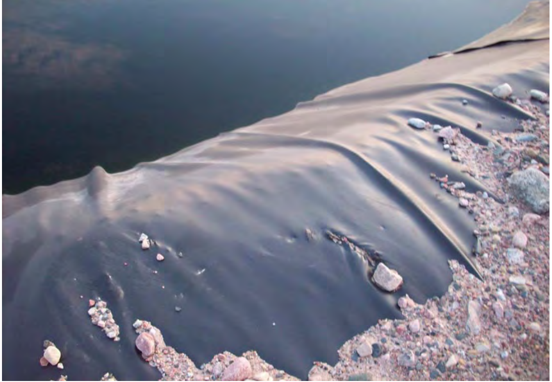
Typical damaged membrane PWSP #1.
