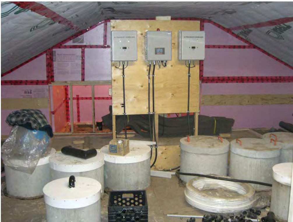
Photo 4: Aeration, final process and UV tanks
