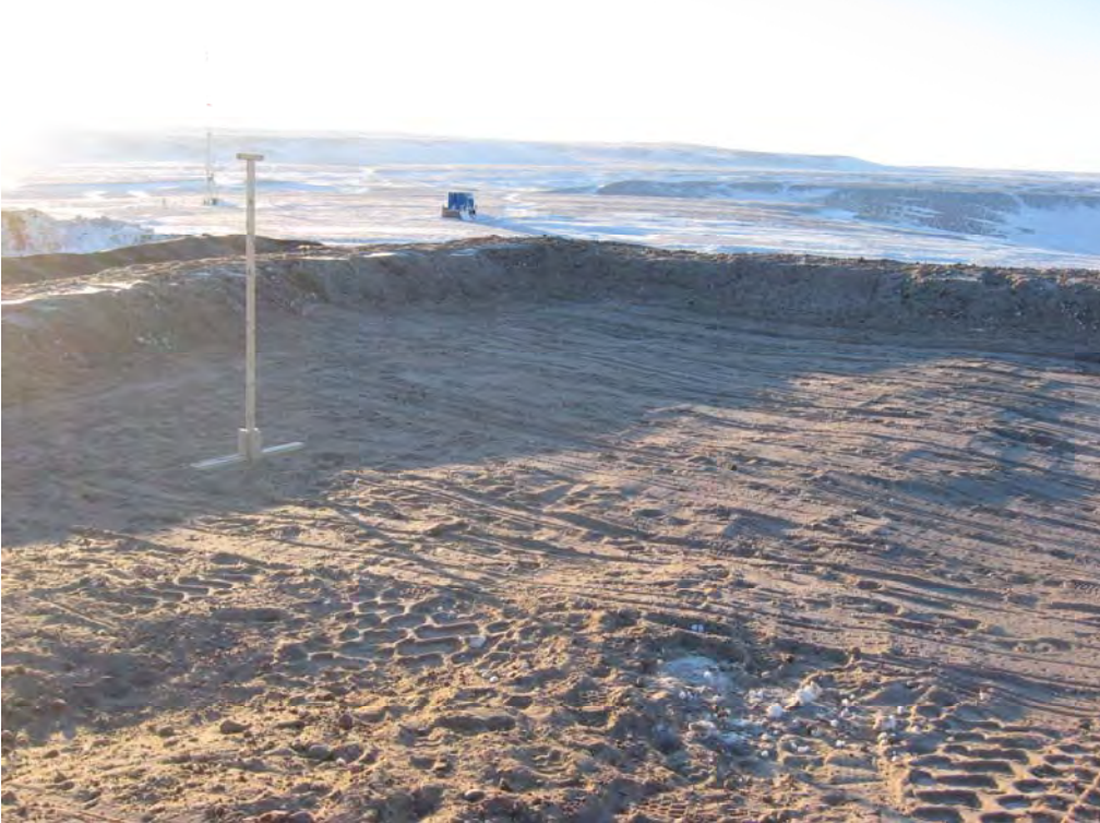
Photo 9: Appropriate amount of cover is being placed over the liner.
