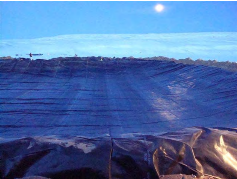
Photo 4: The liner was manufactured and placed as one piece. Thus there was no need for field fusing.
