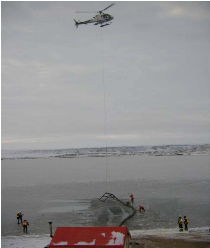
Photo 1: Overview of sewage outfall installation.
