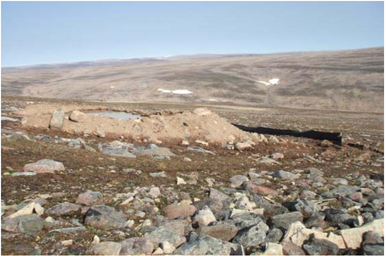
Photo 3: Sump and silt curtain during drilling.
