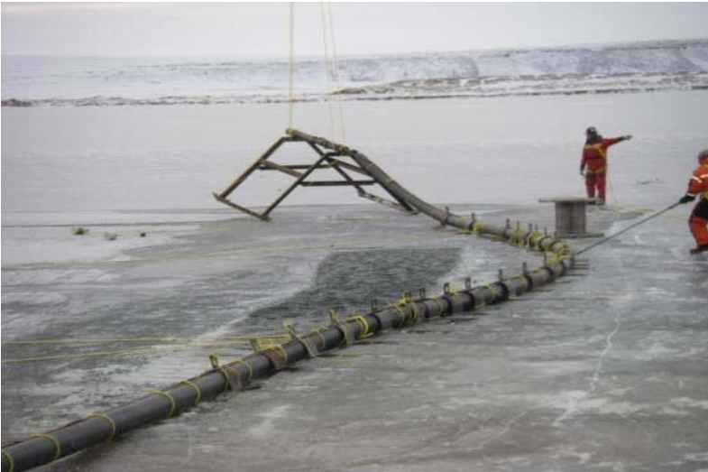
Photo 2: Placing sewage outfall stand on ice.
