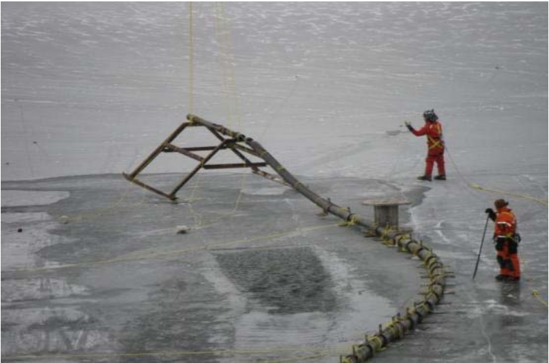
Photo 3: Finalizing positioning on sewage outfall stand.
