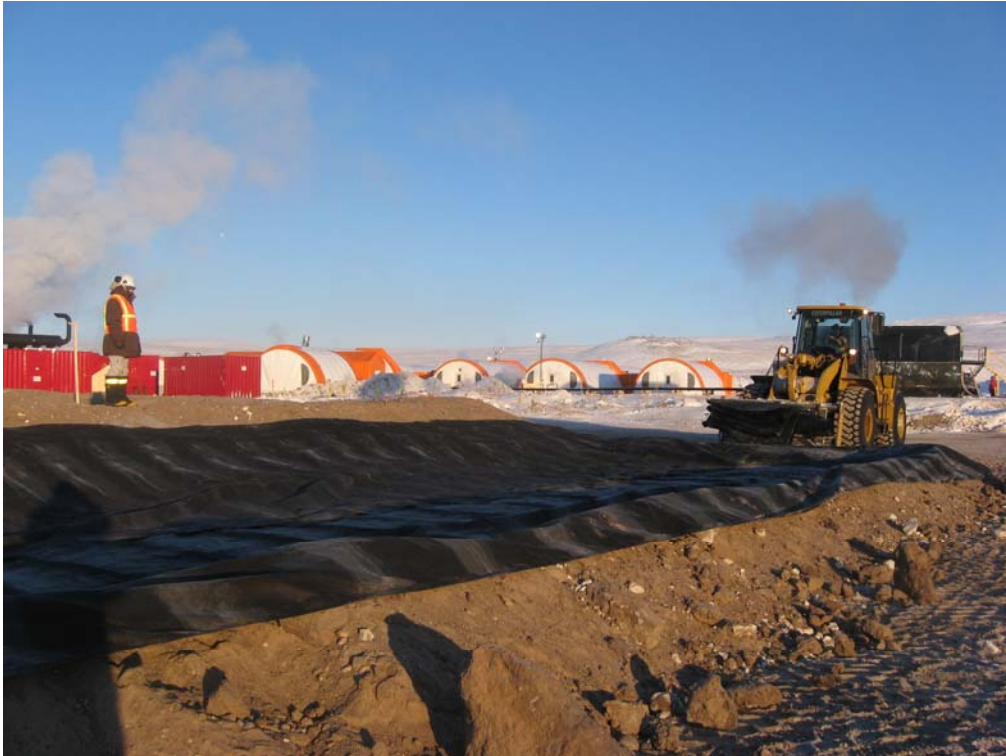
Photo 7: Liner is installed over the slopes. The slopes and the base of the liner will then be protected with appropriate thickness of granular material.
