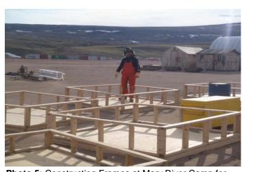
Photo 5: Constructing Frames at Mary River Camp for Portable Containment Berms.
