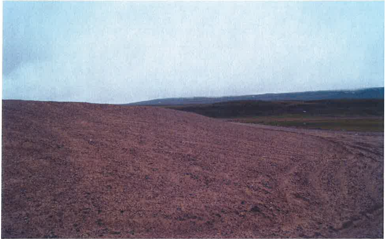
Outside slope of dyke at PWSP No. 3.
