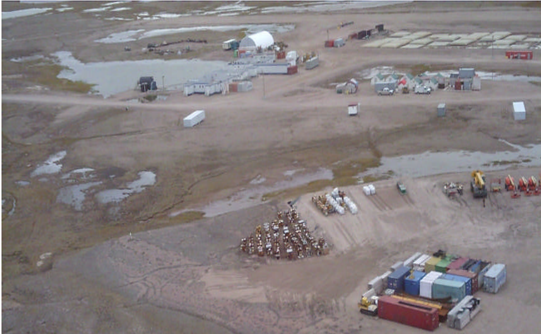
Photo 9 (18) : Milne Inlet Drums, facing southwest
