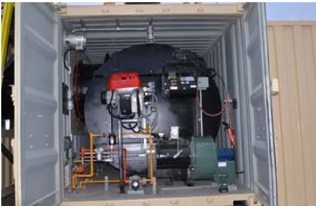
PHOTO 18 Internal view of secondary chamber of new incinerator ልጋሪታል ልጋሪታል ልጋሪታል ልጋሪታል ልጋሪታል
