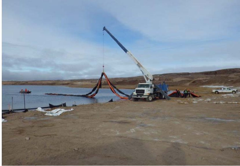
PHOTO 17 Boom deployment and Silt Curtain installation at Camp Lake for Raw Water Jetty
