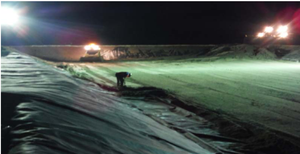
PHOTO 22 Installing arctic liner at Steel Tank Bulk Fuel Storage Facility engineering containment structure August 2013
