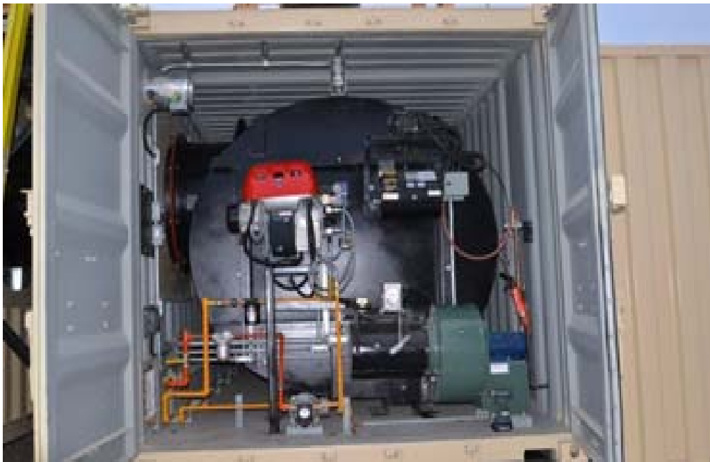
PHOTO 18 Internal view of secondary chamber of new incinerator ልጋላሙር ርዕሳ ለክር ለሮኪልኤር ወርሻ ልብረብልኤ
