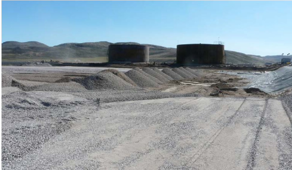
PHOTO 11 Construction of Steel Tank Bulk Fuel Storage Facility Pad (alternate view) July 2013
