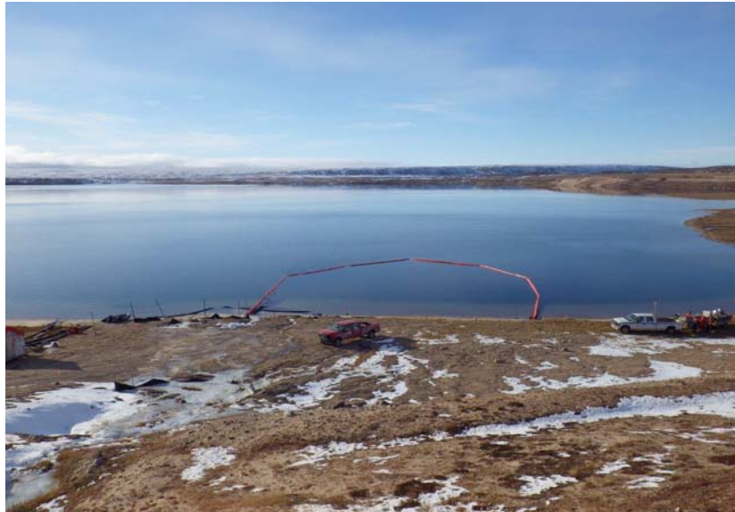
PHOTO 18 Mine Site Raw Water Jetty Silt Curtain at Camp Lake
