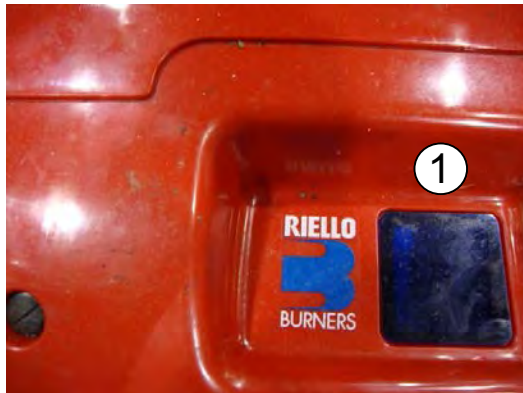
1. Primary Burner Inspection Window
