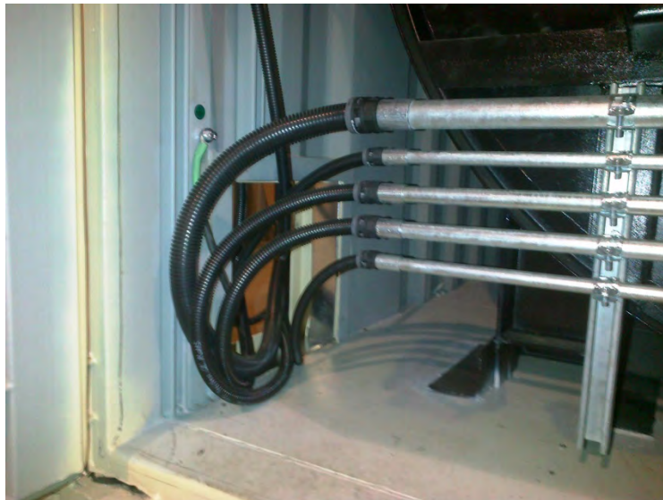
Flexible conduit in Container 2 (secondary chamber)
