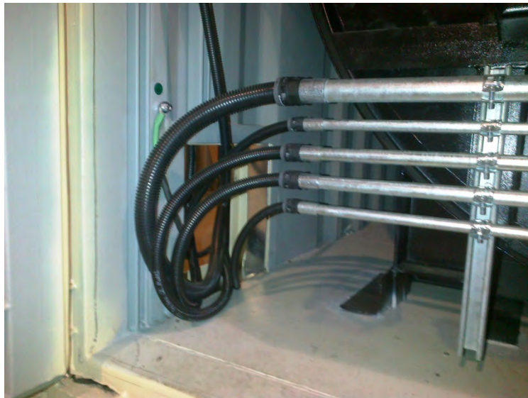
Flexible conduit in Container 2 (secondary chamber)
