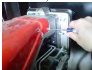
Secondary Burner has 4 screws (2 on each side)
