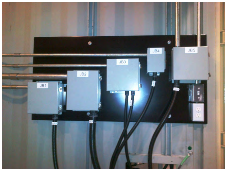
Junction Boxes in container 3 (control container)
