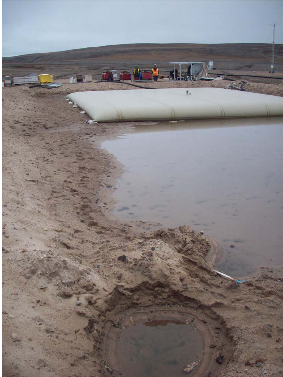
Generator Fuel Containment Cell (shows test pit to establish membrane elevation)
