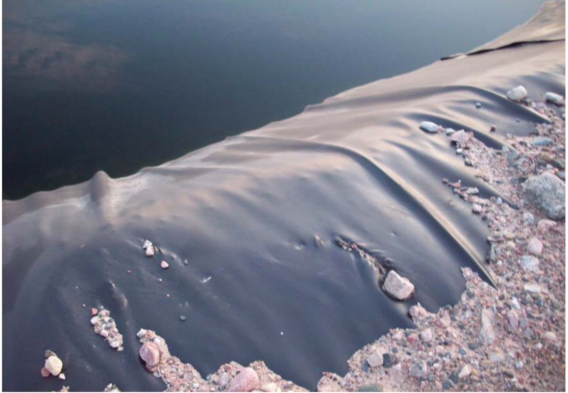
Typical damaged membrane PWSP #1.
