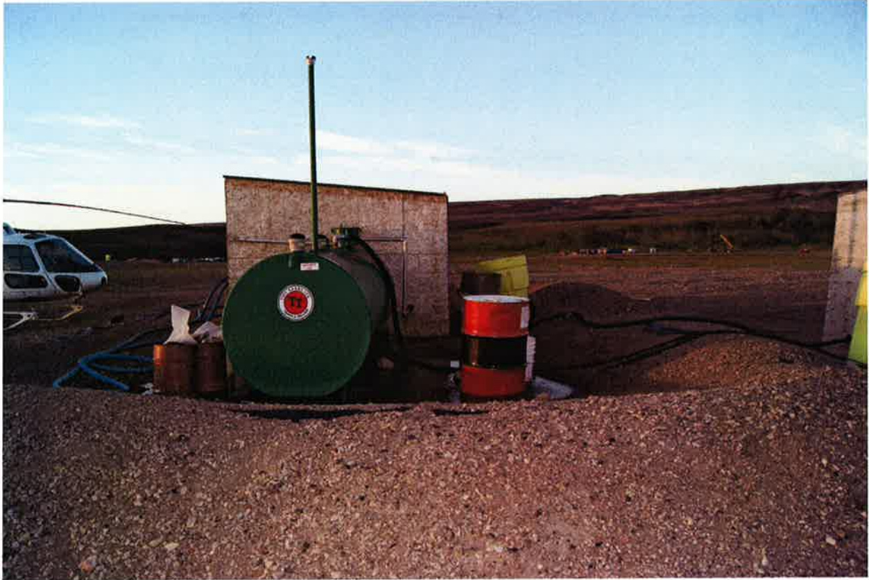
Helicopter Fuel Tank Containment – Mary River
