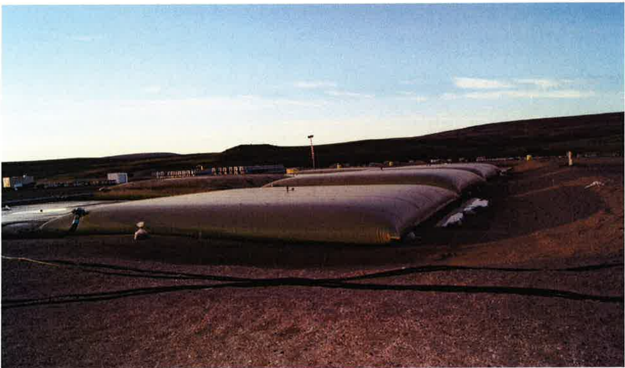
Bulk Fuel Storage Facility Containment – Mary River
