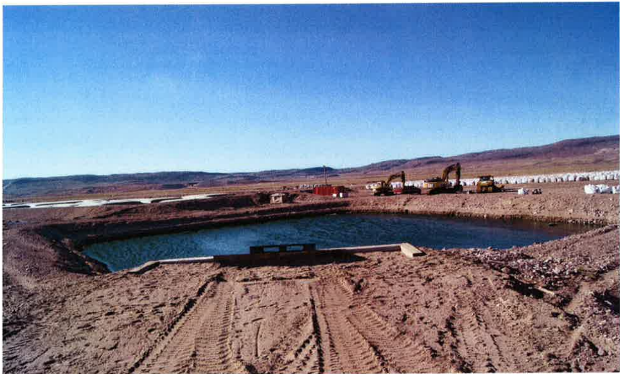
Polishing/Waste Stabilization Pond – Milne Inlet.
