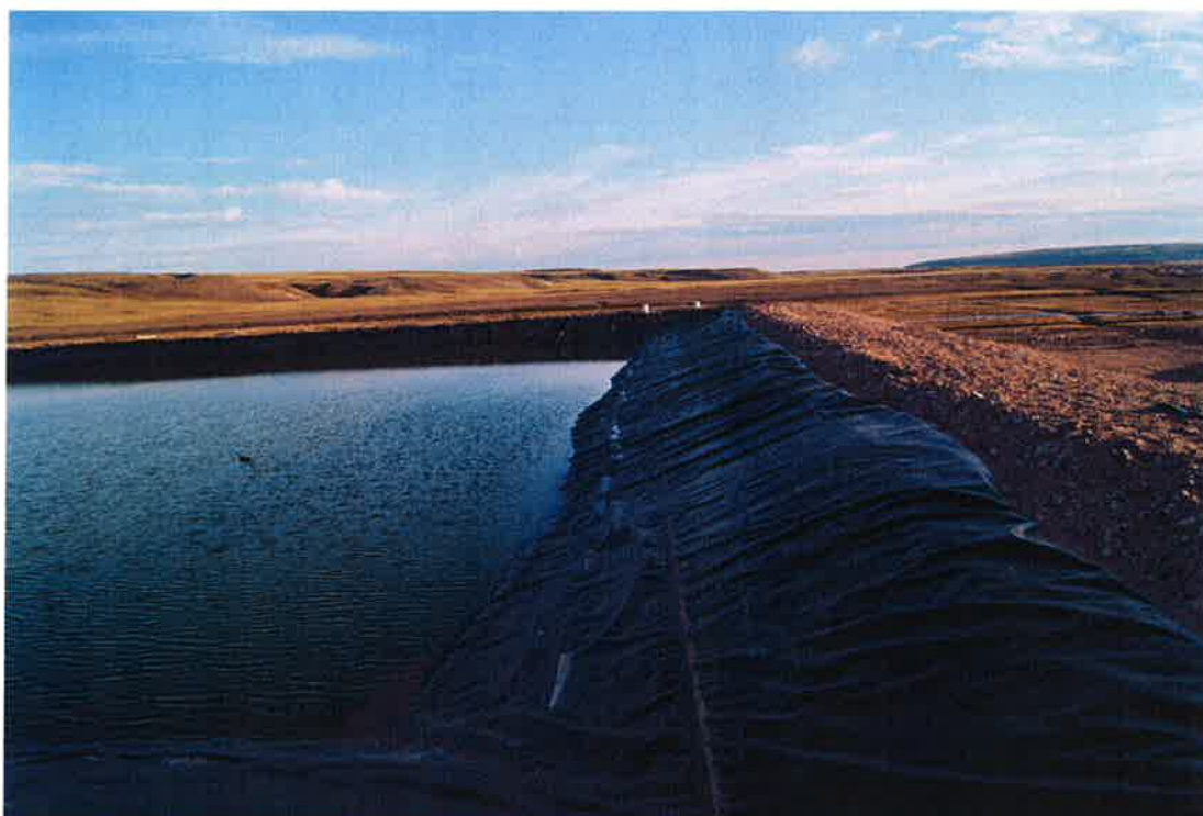
Typical dyke structure PWSP #2 – Mary River
