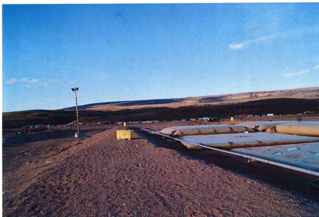
Typical dyke – Bulk Fuel Containment – Mary River
