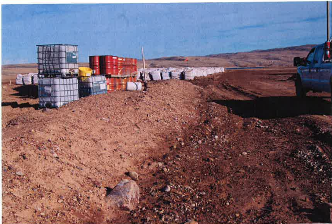
Oil and Antifreeze Containment – Milne Inlet
