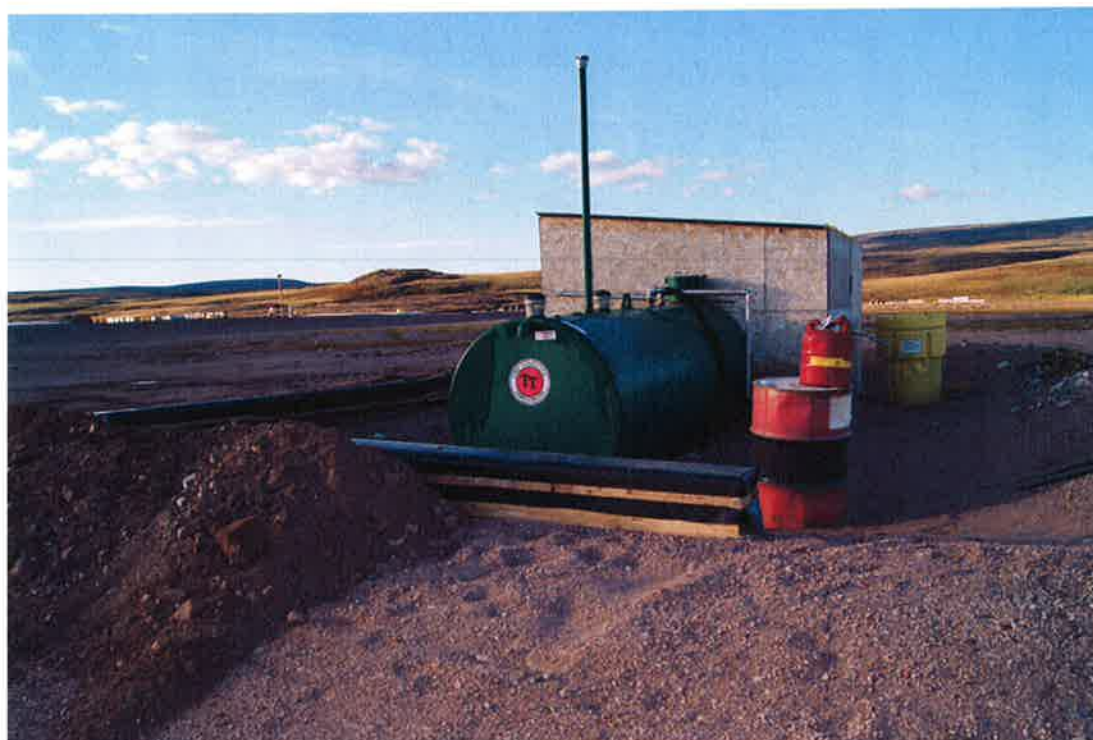
Helicopter Fuel Cell Containment – curb sits above dyke – Mary River
