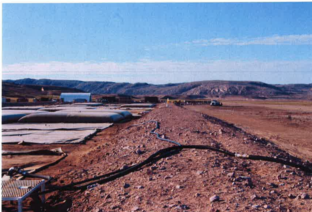
Typical dyke Milne Inlet Bulk Fuel Containment
