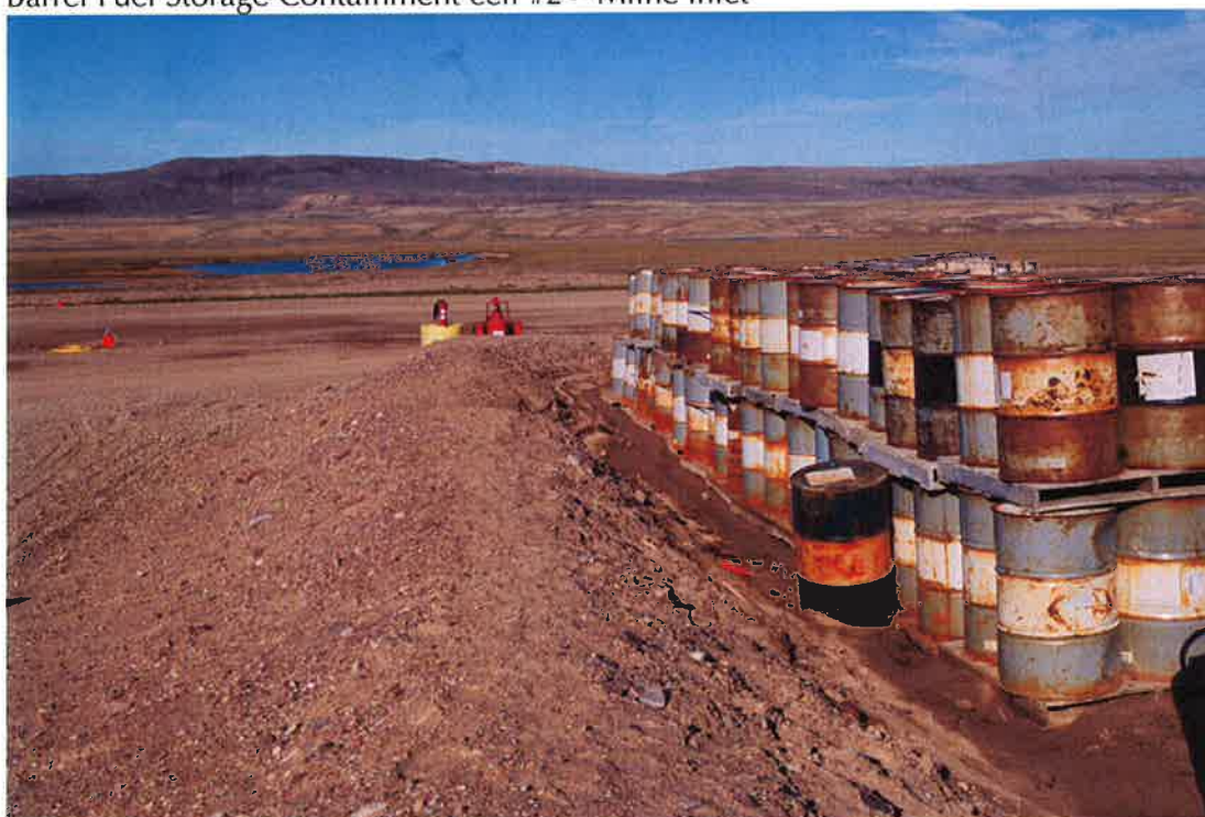
Typical Dyke Barrel Fuel Containment – Milne Inlet
