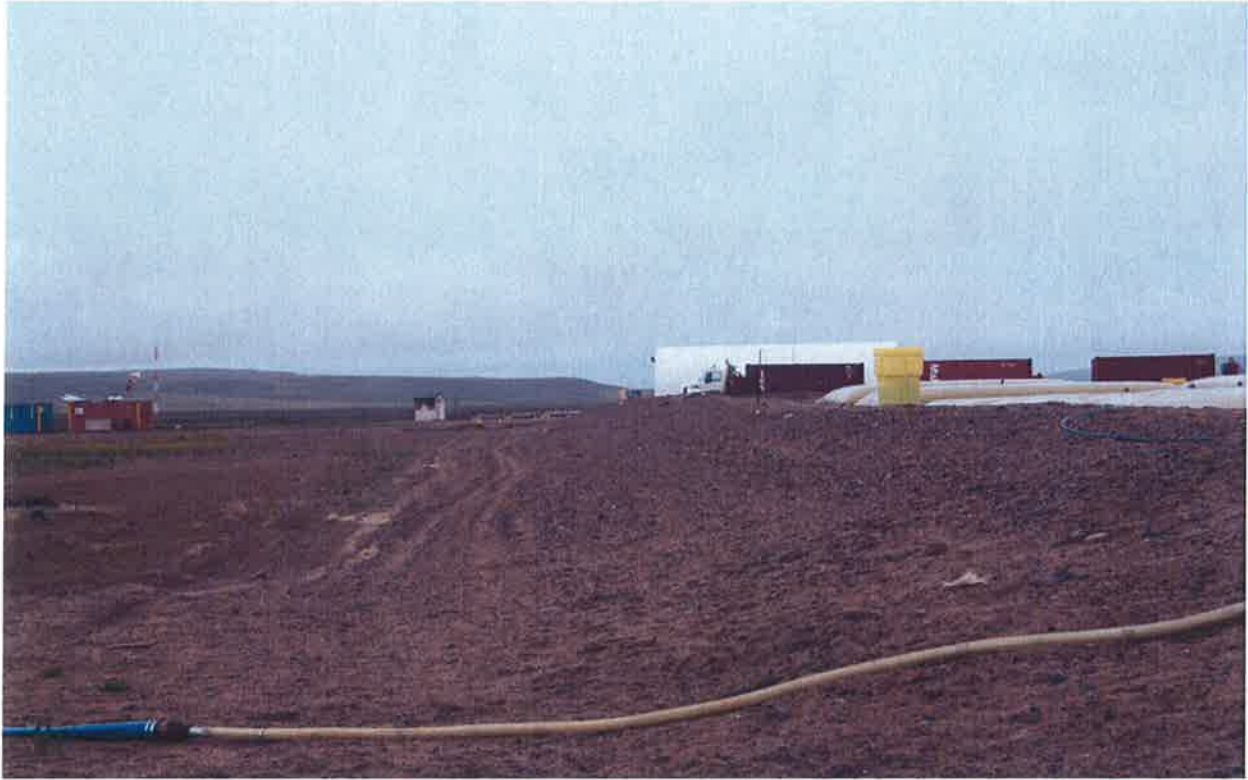
Outside slope of dyke at the Bulk Fuel Storage Facility containment.
