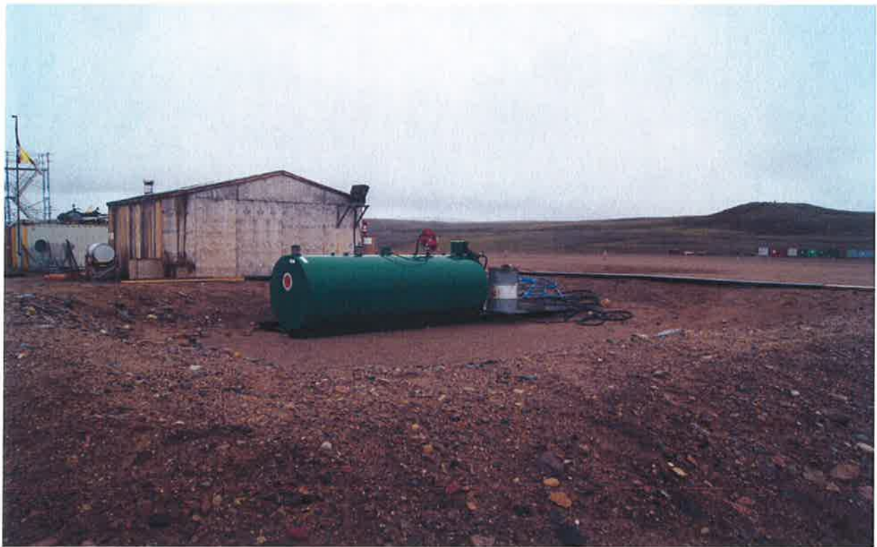
Jet Fuel Tank and Pump Containment.
