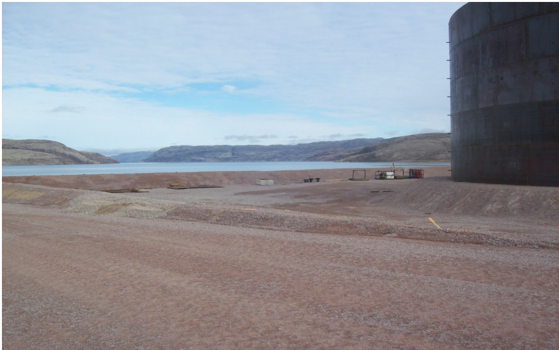
Exterior of dyke – Fuel Tank Farm
