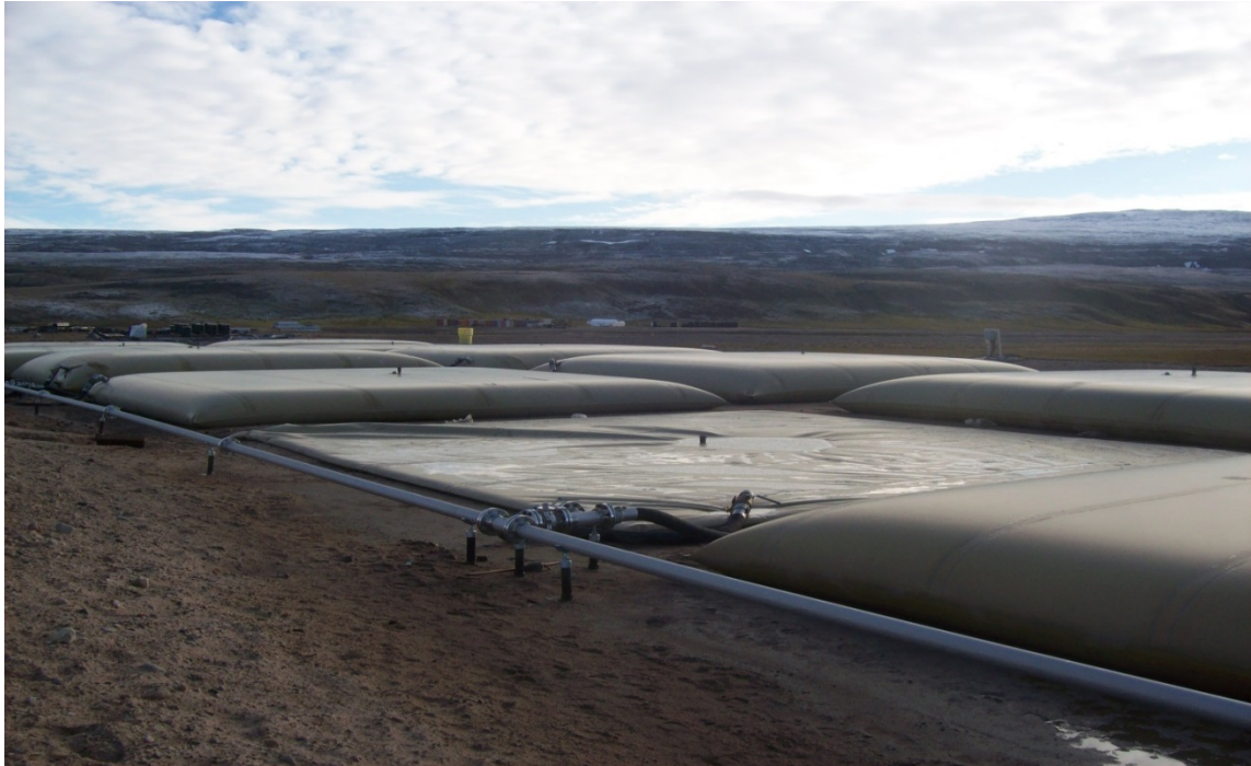
Interior of Bulk Fuel Storage Containment Shows trapped water in containment.
