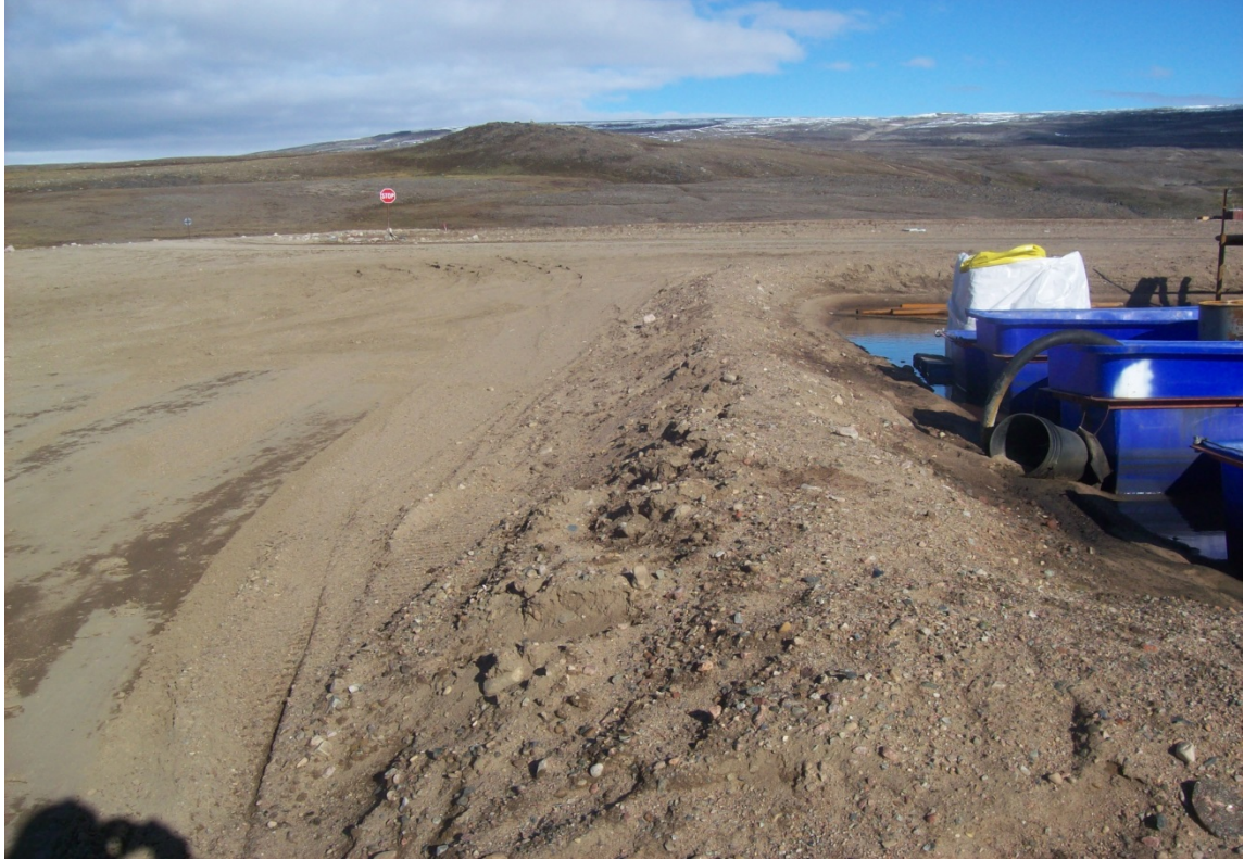
Dyke at Waste Oil Storage.
