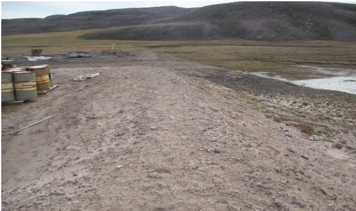
Hazardous Waste Storage dyke.
