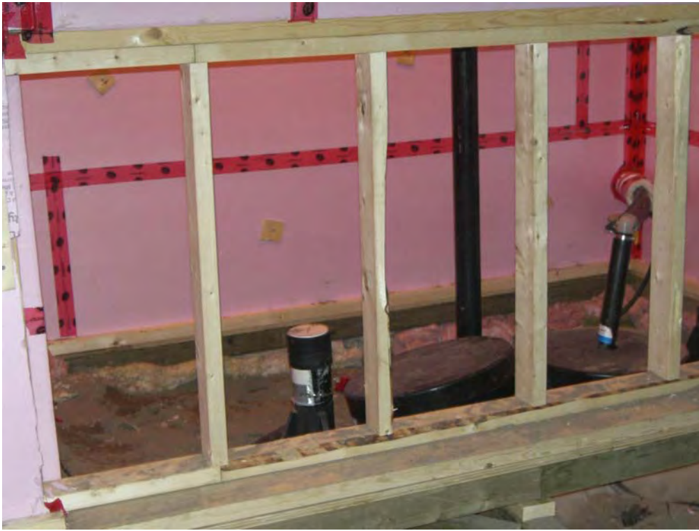
Photo 5: Final pumping chamber going to the PWSP
