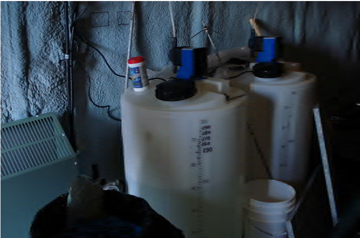
Photo 4: Alum & Sodium Bicarbonate Tanks
