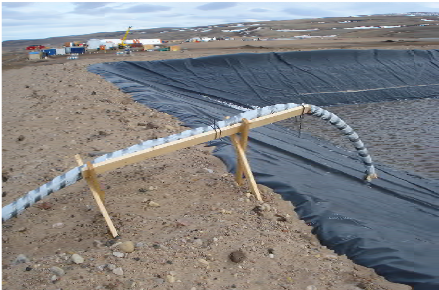
Photo 9: View of the PWSP #1 with discharge (during construction )
