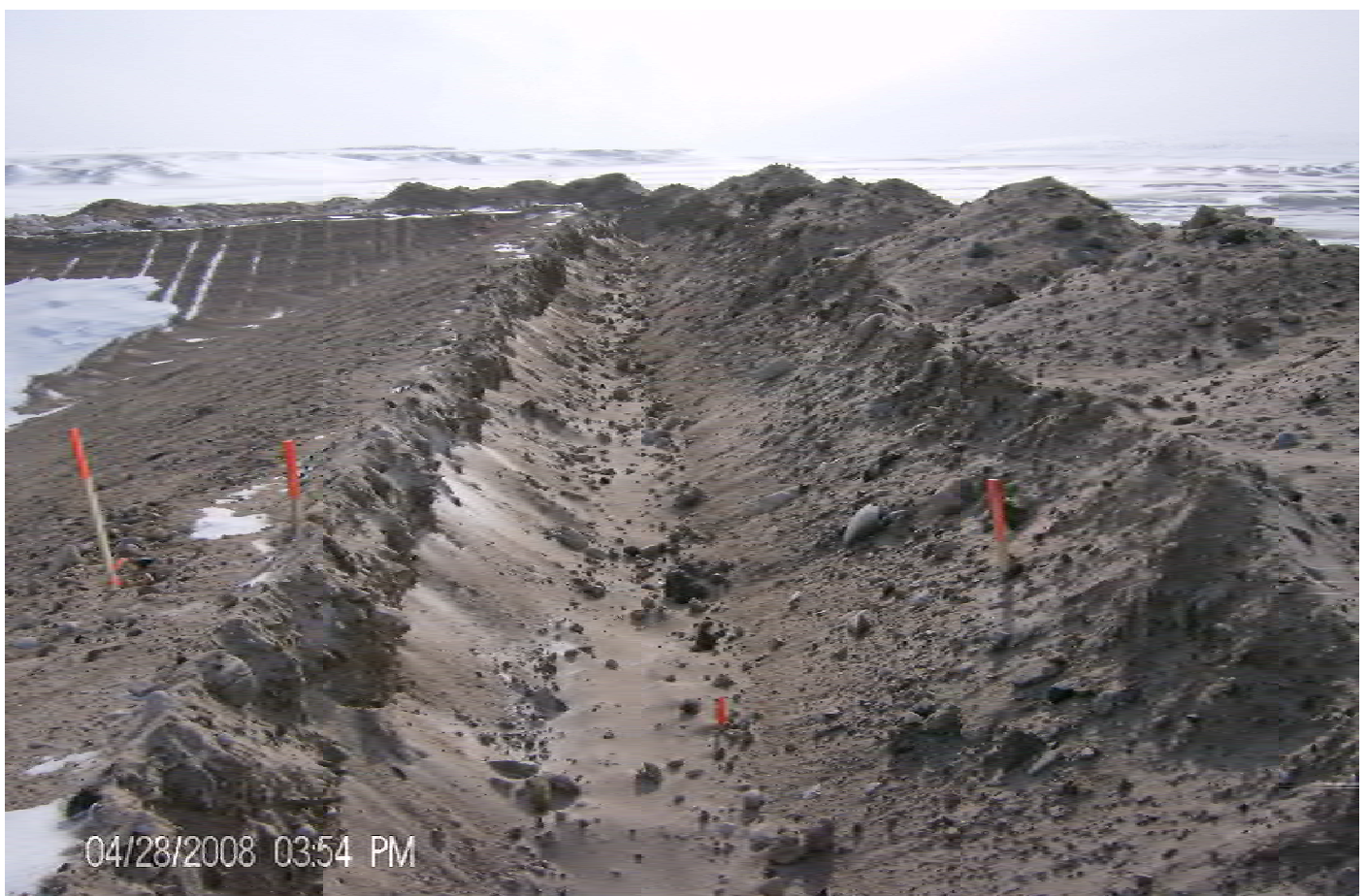
Photo 12: View of the PWSP #2 trench for liner during construction )
