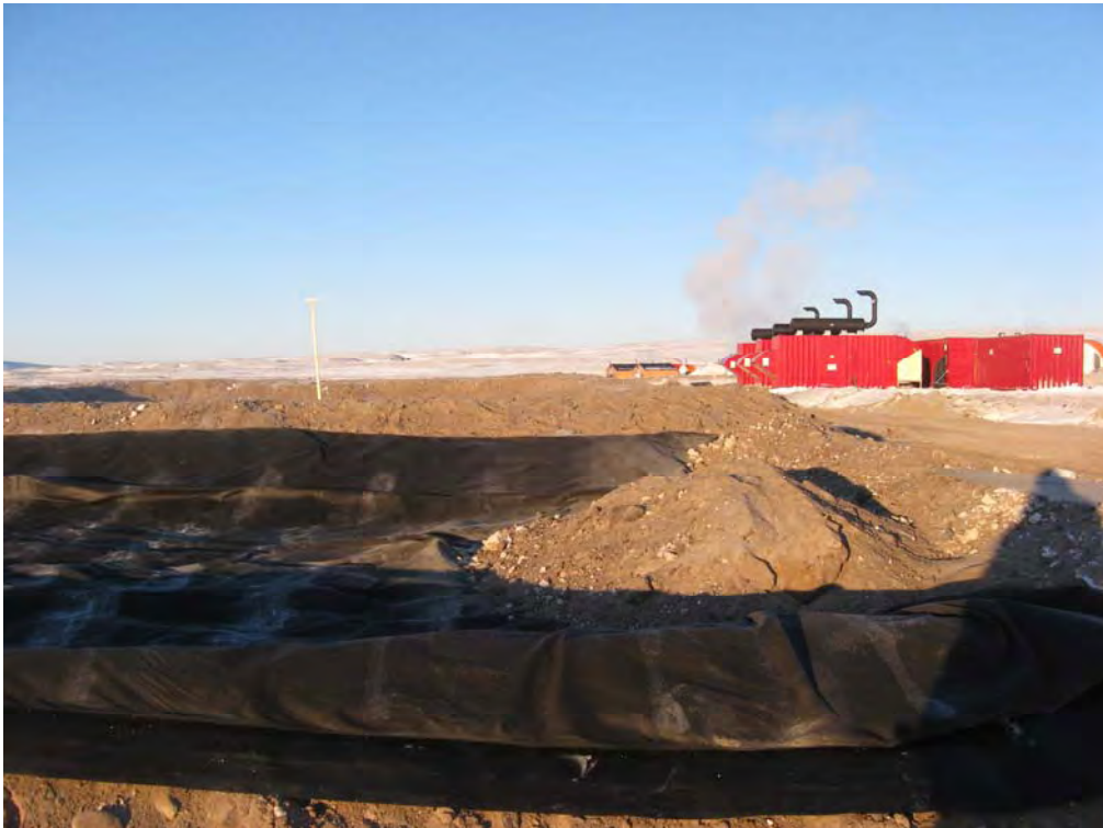
Photo 8: Granular material is being placed over the liner.
