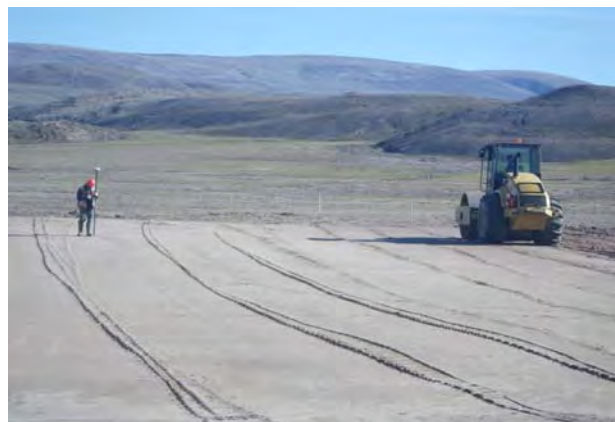
Lift two being compacted and elevation being checked by surveyor
