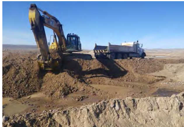
345 Excavator loading Haul Truck at Km2 Borrow Pit
