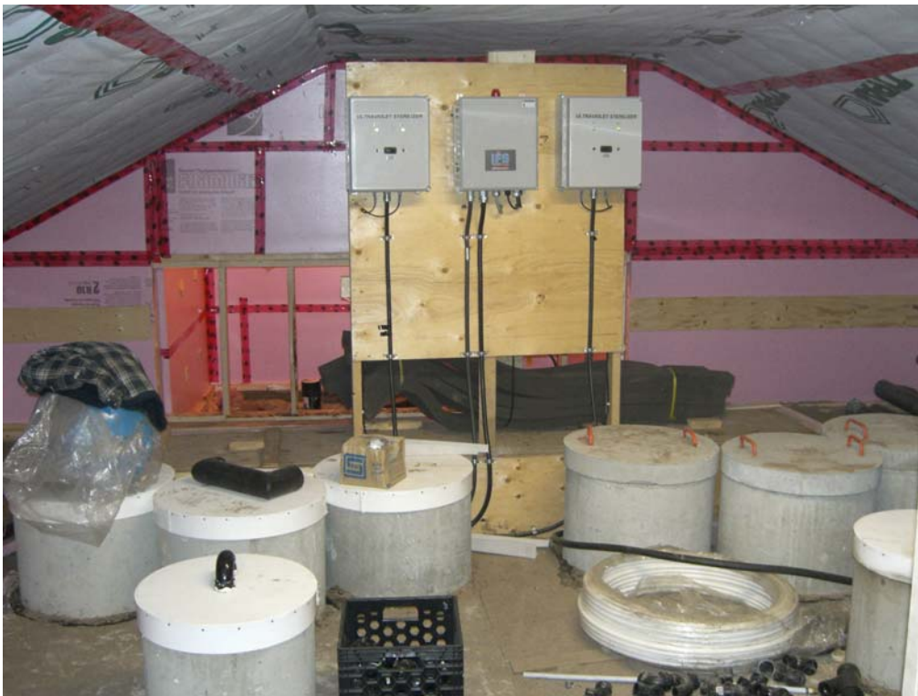
Photo 4: Aeration, final process and UV tanks
