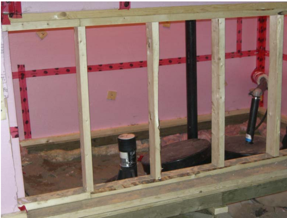
Photo 5: Final pumping chamber going to the PWSP
