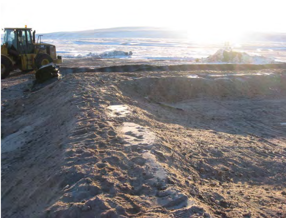
Photo 4: The slopes and the base are ready for the installation of the liner.
