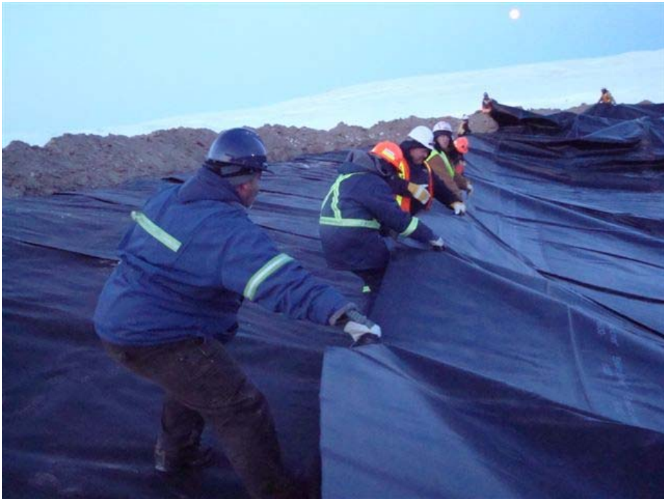
Photo 2: Crew is installing the liner at PWSP #3
