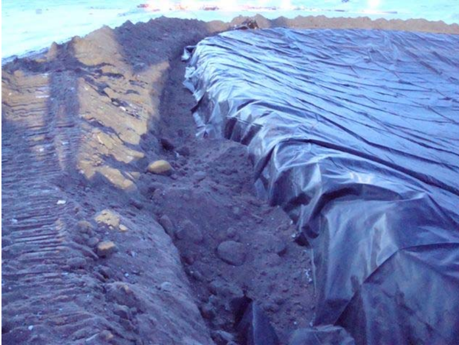
Photo 3: The liner is anchored in the trench at the top of the berm
