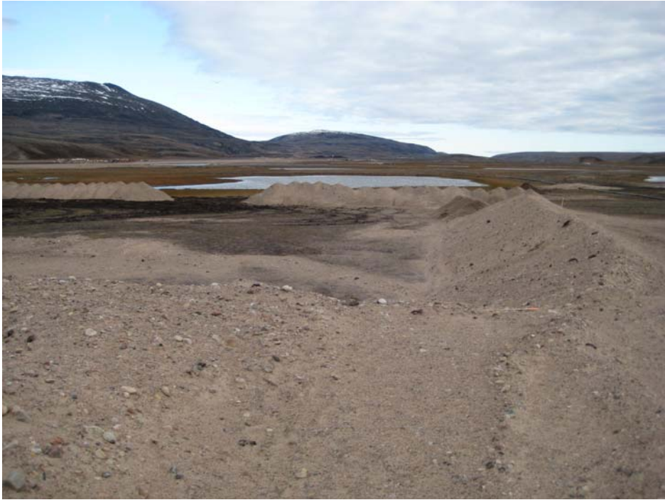
Photo 1: Material has been brought to the PWSP #3 site for placement and berm construction
