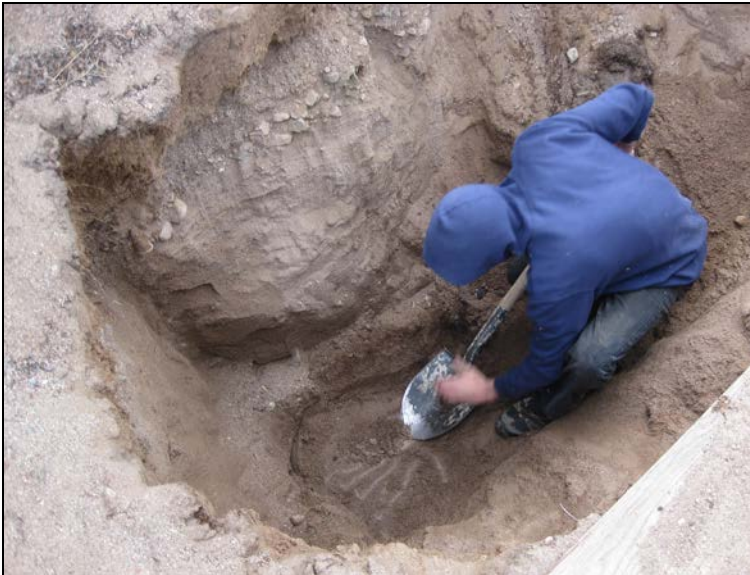
Figure 4: Scrapping Non-Contaminated Sands from Upper Permafrost Horizon
