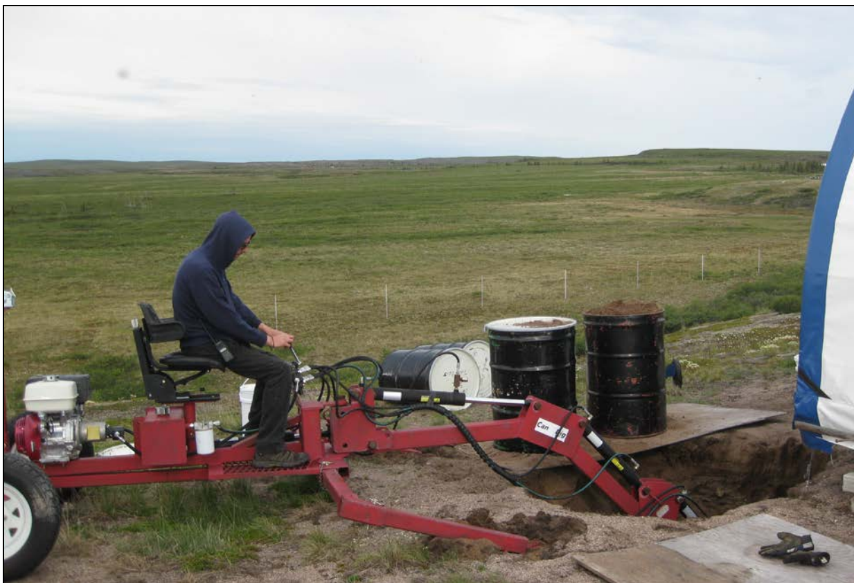
Figure 1: Can-Dig Excavator Removal of 4 Drums of Contaminated Soil to Permafrost - 2015
