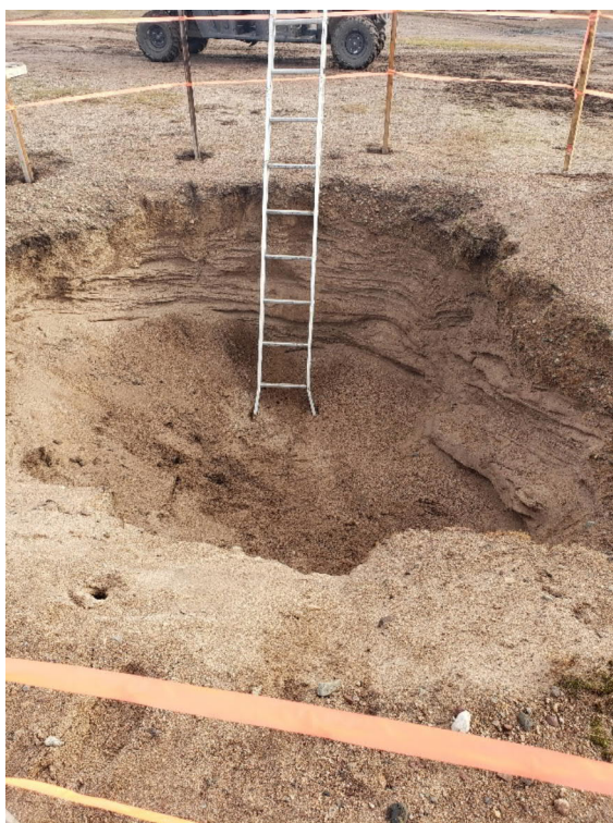
Figure 10: Site of Spill File 2023-146, collapsed sidewalls cordoned off for winter.
