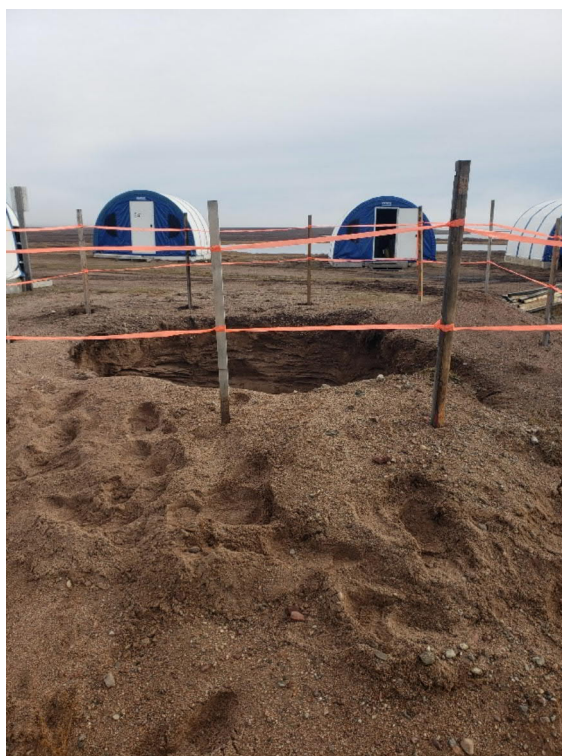
Figure 10: Site of Spill File 2023-146, collapsed sidewalls cordoned off for winter.
