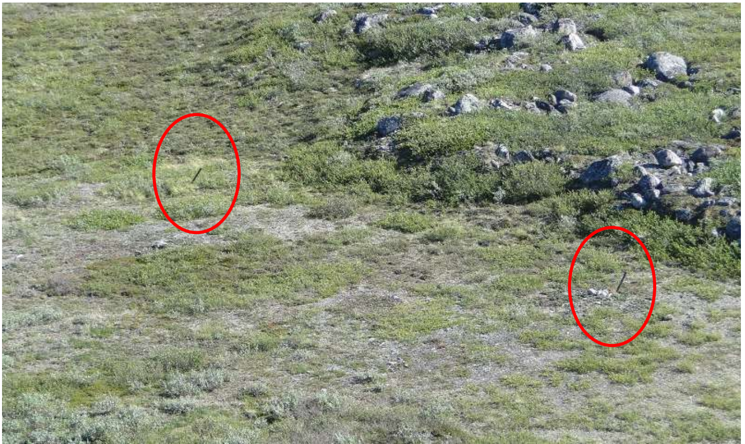
Figure 7. Drill sites appear clean, but casing needs to be removed or cut off as per licence.
