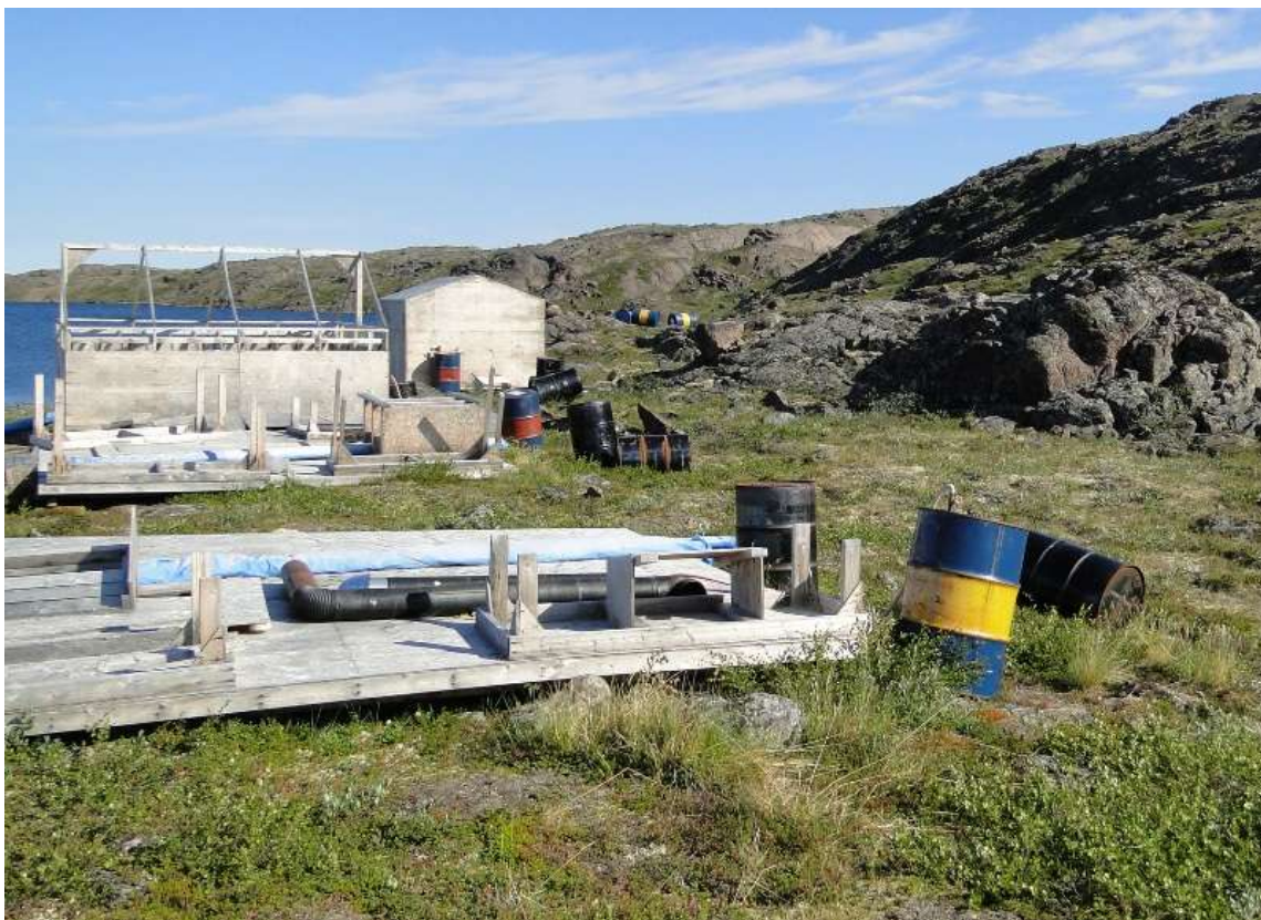
Figure 9. No secondary containment was used on-site; many barrels have leaked over time.
