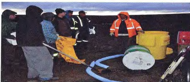
Hazardous material boom placed around the spill.
