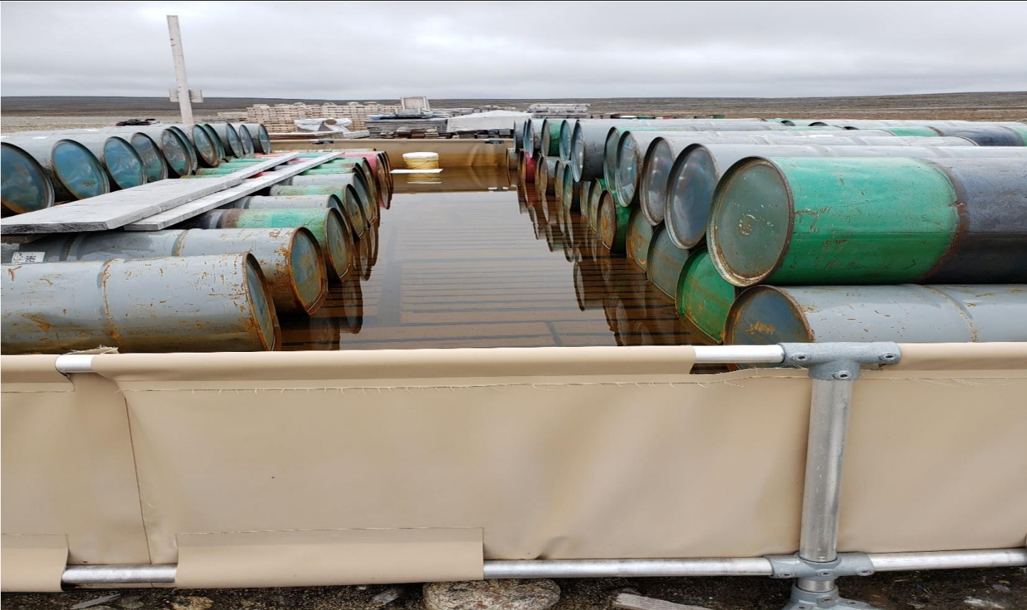
Description: fuel cache 3 in secondary containment. Liquid contained in berm. Leak on the carbon filter observed.
