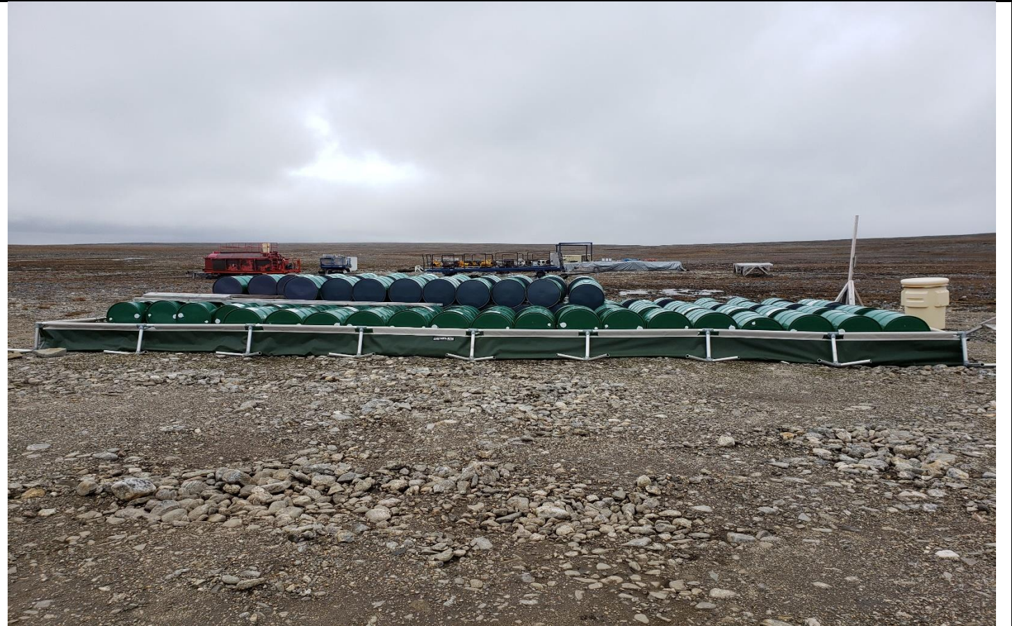
Description: Fuel Cache – Approximately 60 drums of fuel in secondary containment, spill kit observed.
