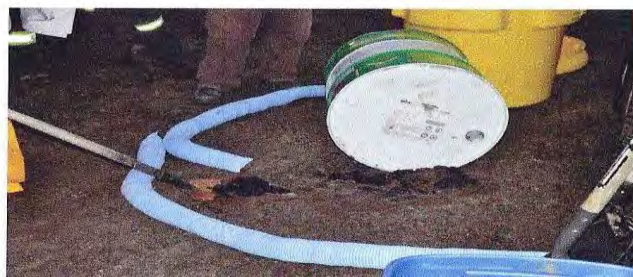
Contaminated soil shovelled into spill kit.
