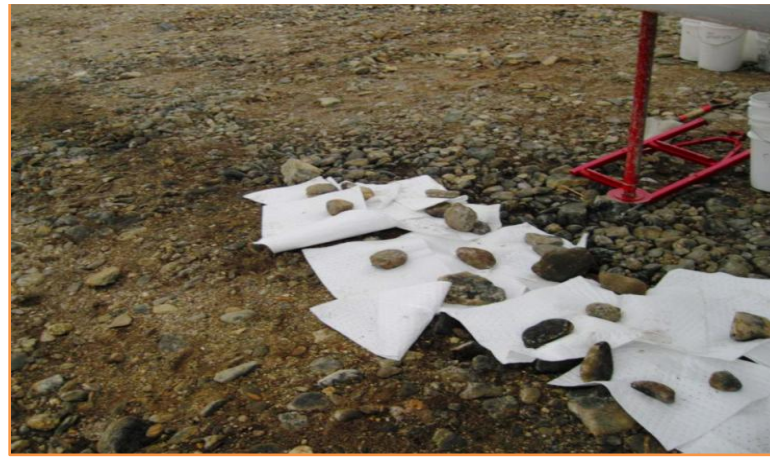
Left: Spill-kit drum, pails captured 25L immediately. Above: Spill pads on fuel trail.
