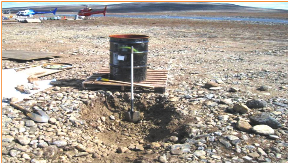
Above: Cobbles, rocks and gravelly, silty soil was shovelled out and placed in containers. Right: Peregrine staff backfilled area with clean native material from the apron area.
