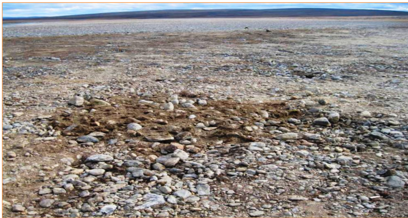
Above: Cobbles, rocks and gravelly, silty soil was shovelled out and placed in containers. Right: Peregrine staff backfilled area with clean native material from the apron area.
