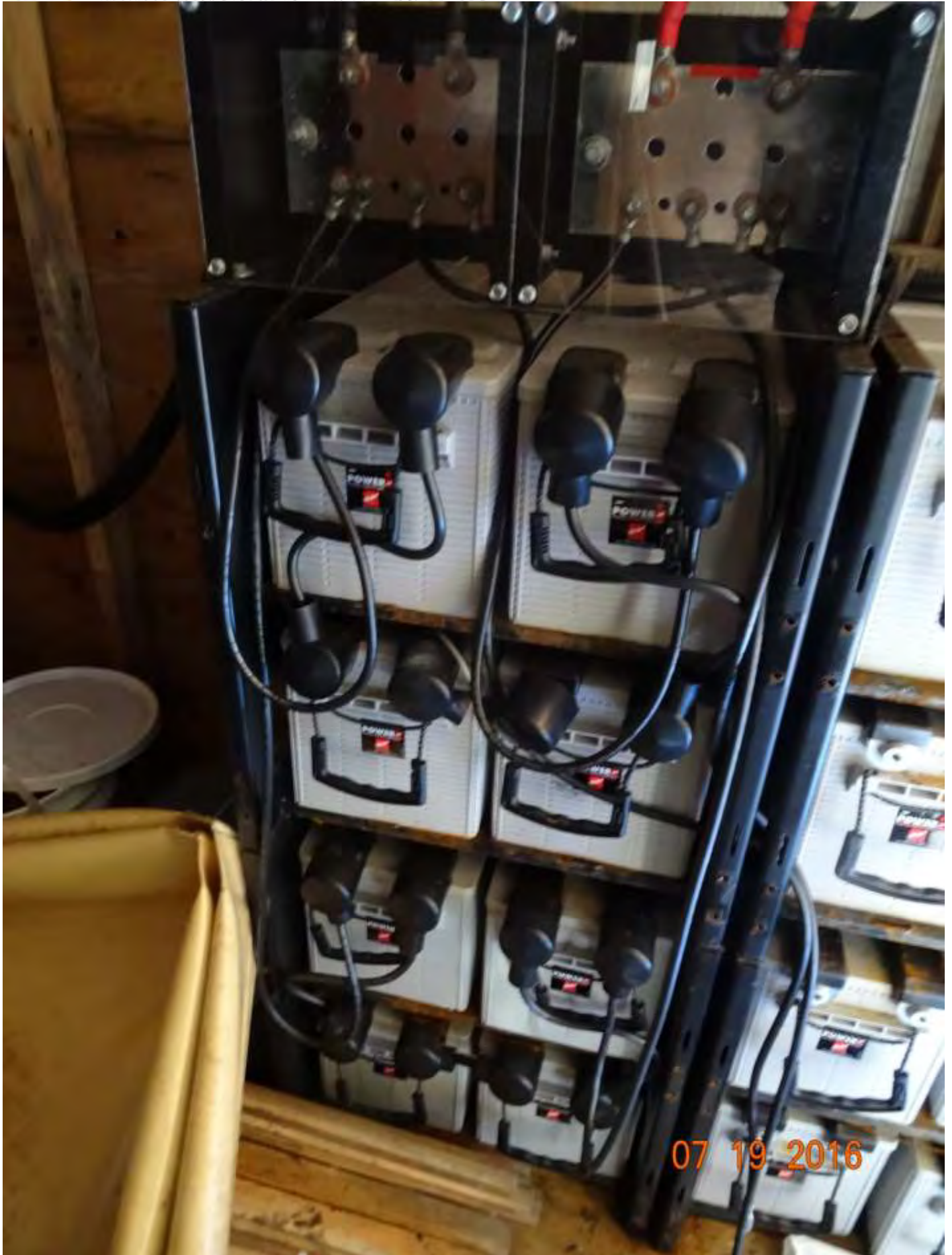
Photo 31: Batteries for Solar Panels
