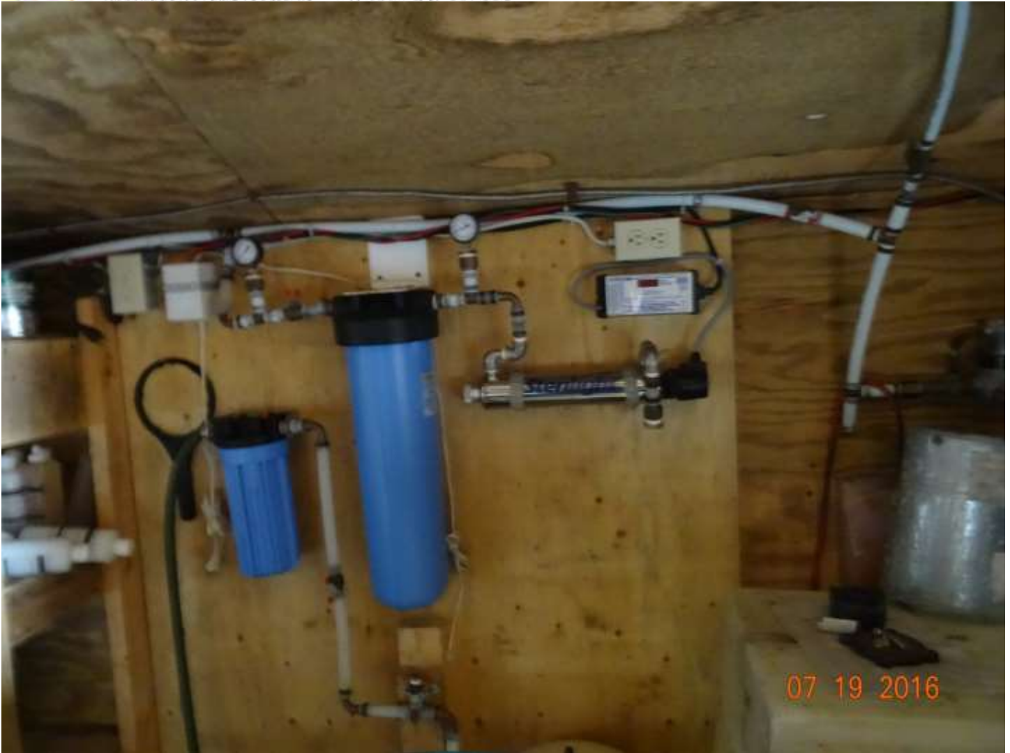
Photo 38: Water treatment system
