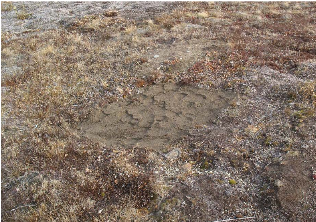
Photo 4 : September 2013 - Sump filled in, levelled, and scarred to promote regrowth.
