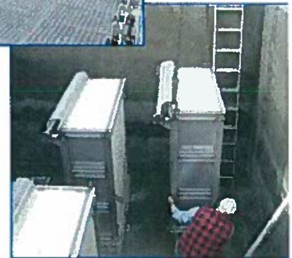
Installing the MBR units.
