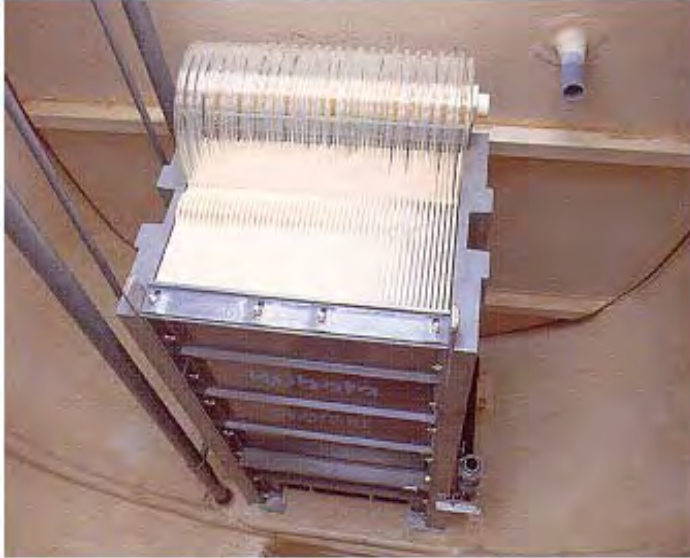
Figure 4. Photo of a membrane module, composed of approximately 100 membranes, connected to a collection manifold by rubber tubes.
