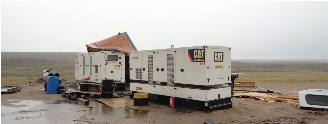
Figure 12 – Demolished Power Generation Shack
