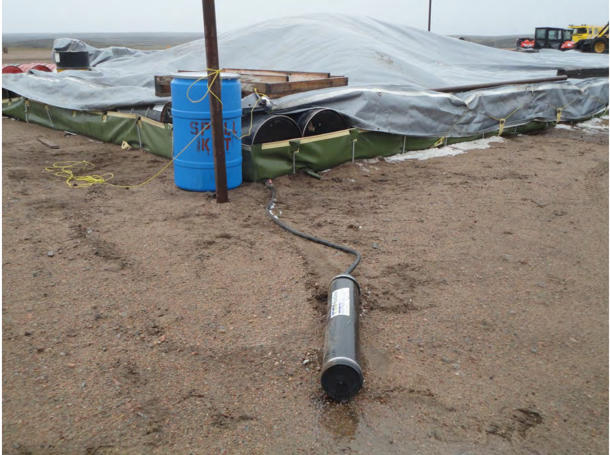
Figure 6 – Rain Drain filters attached to drain water from berm
