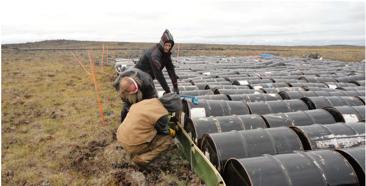
Figure 20 – Replacing damaged support brackets on berm 3 at Three Bluffs.
