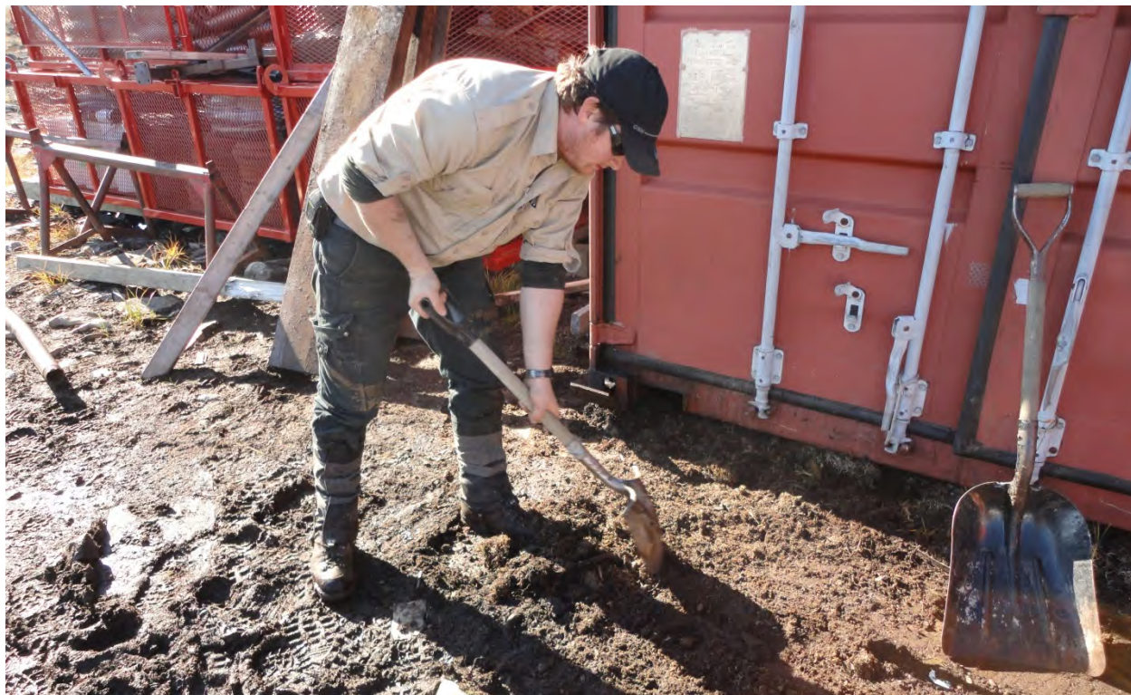
Figure 26 – Removing contaminated soil from door of red sea container.
