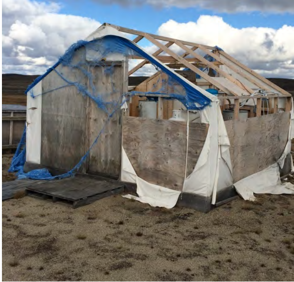
Figure 33 – Repaired tent at Bullion Camp.
