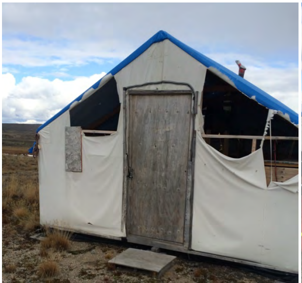
Figure 34 – Repaired tent canvas at Bullion Camp.
