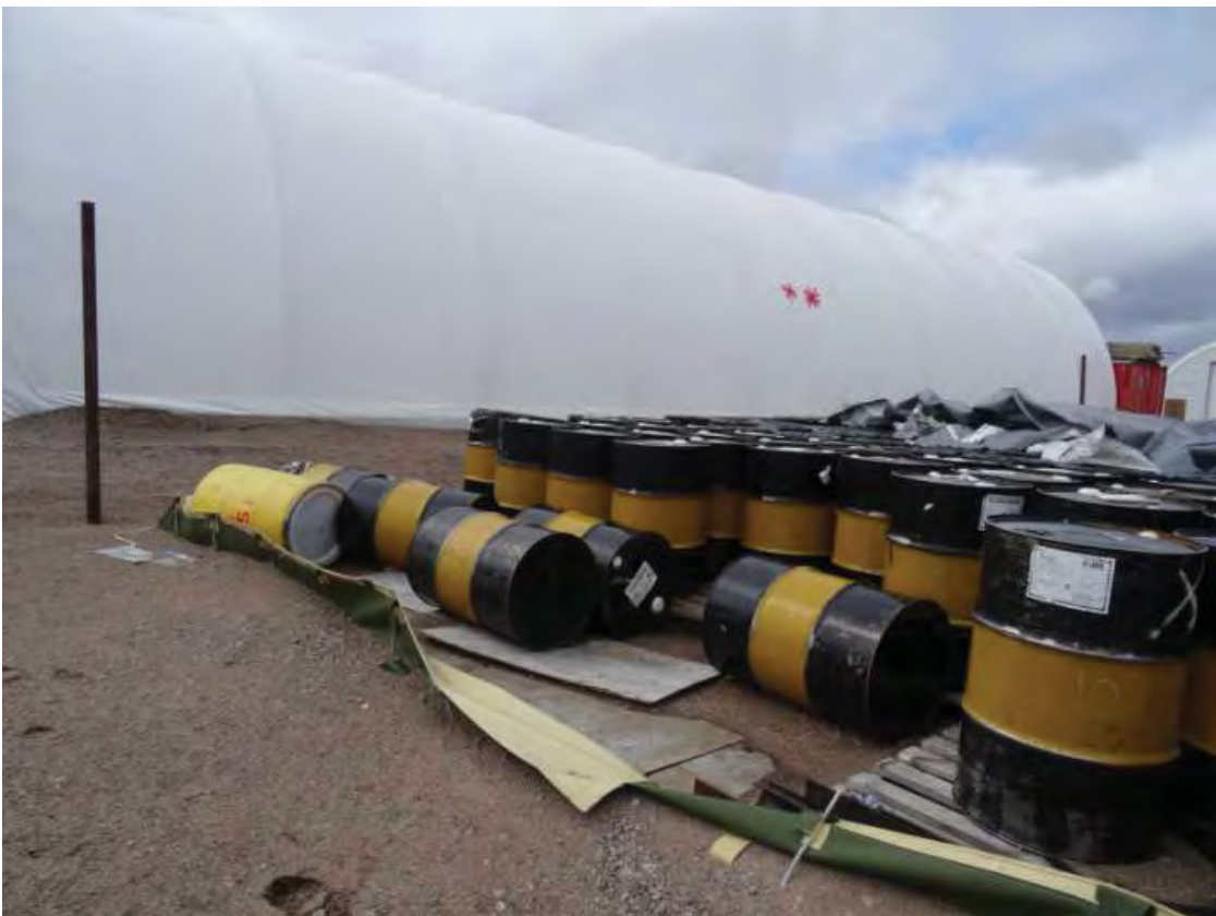
Figure 10. Hayes berm collapsed.
