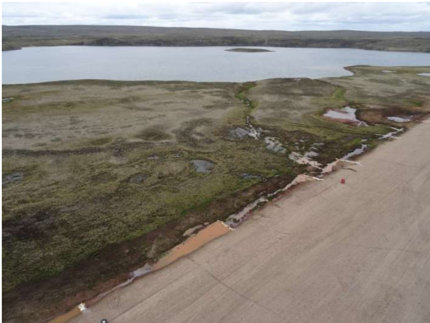
Figure 16. Pooling/ponding on the side of the airstrip; sediment evident in water flowing down-slope.
