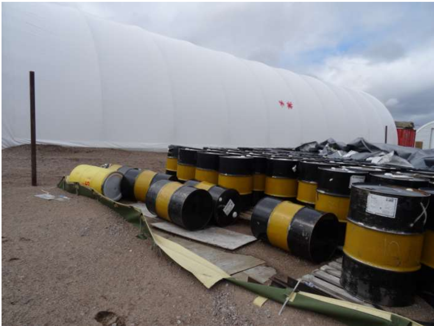
Figure 10. Hayes berm collapsed.
