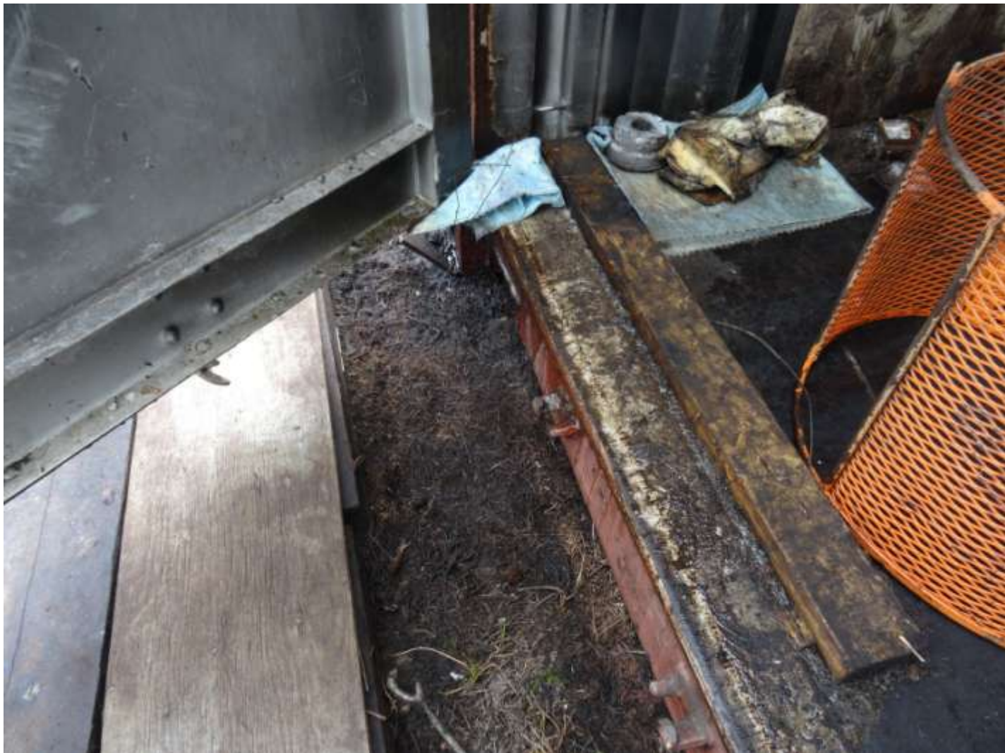
Figure 27. Sea-can leaking oil-contaminated water; there is water coming into the sea-can and flowing through.
