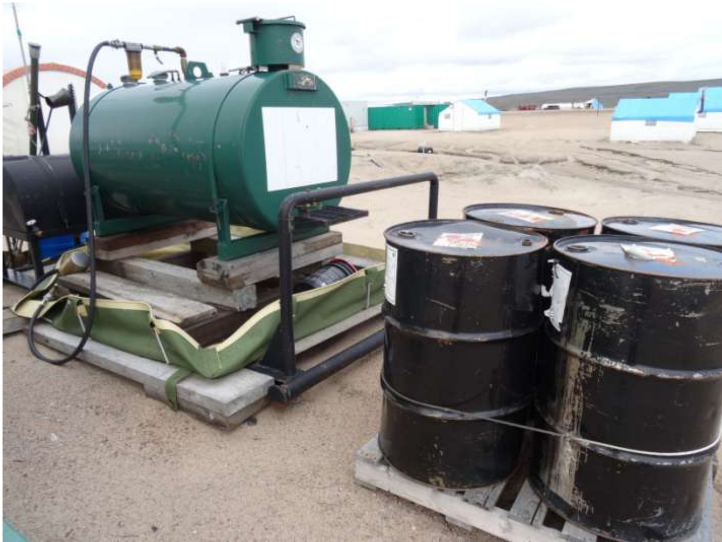
Figure 21. Barrels out of containment at the incinerator.
