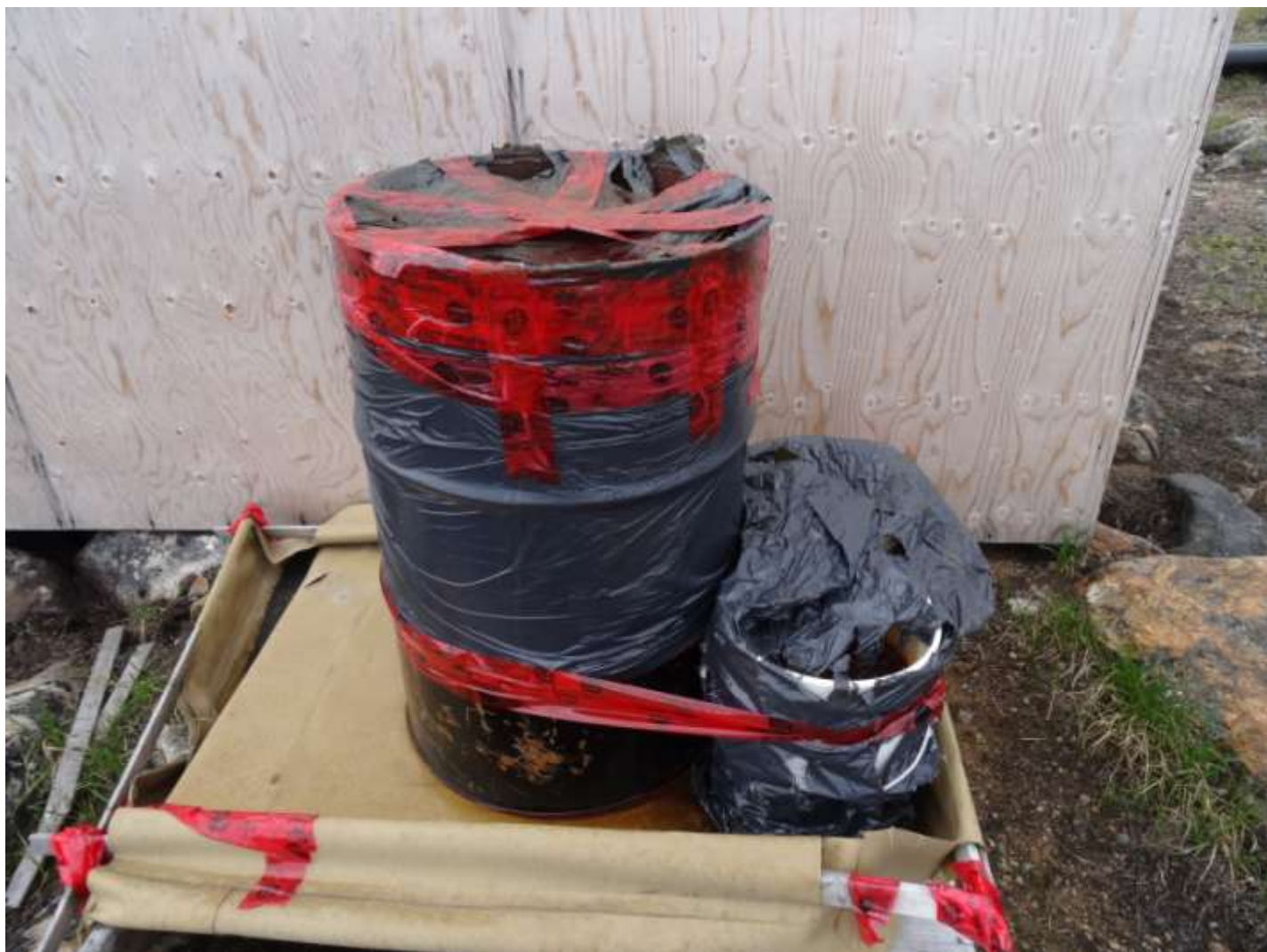
Figure 29. Covered drums of assumedly contaminated material at the boiler. Berm is destroyed, and barrel contents are exposed.
