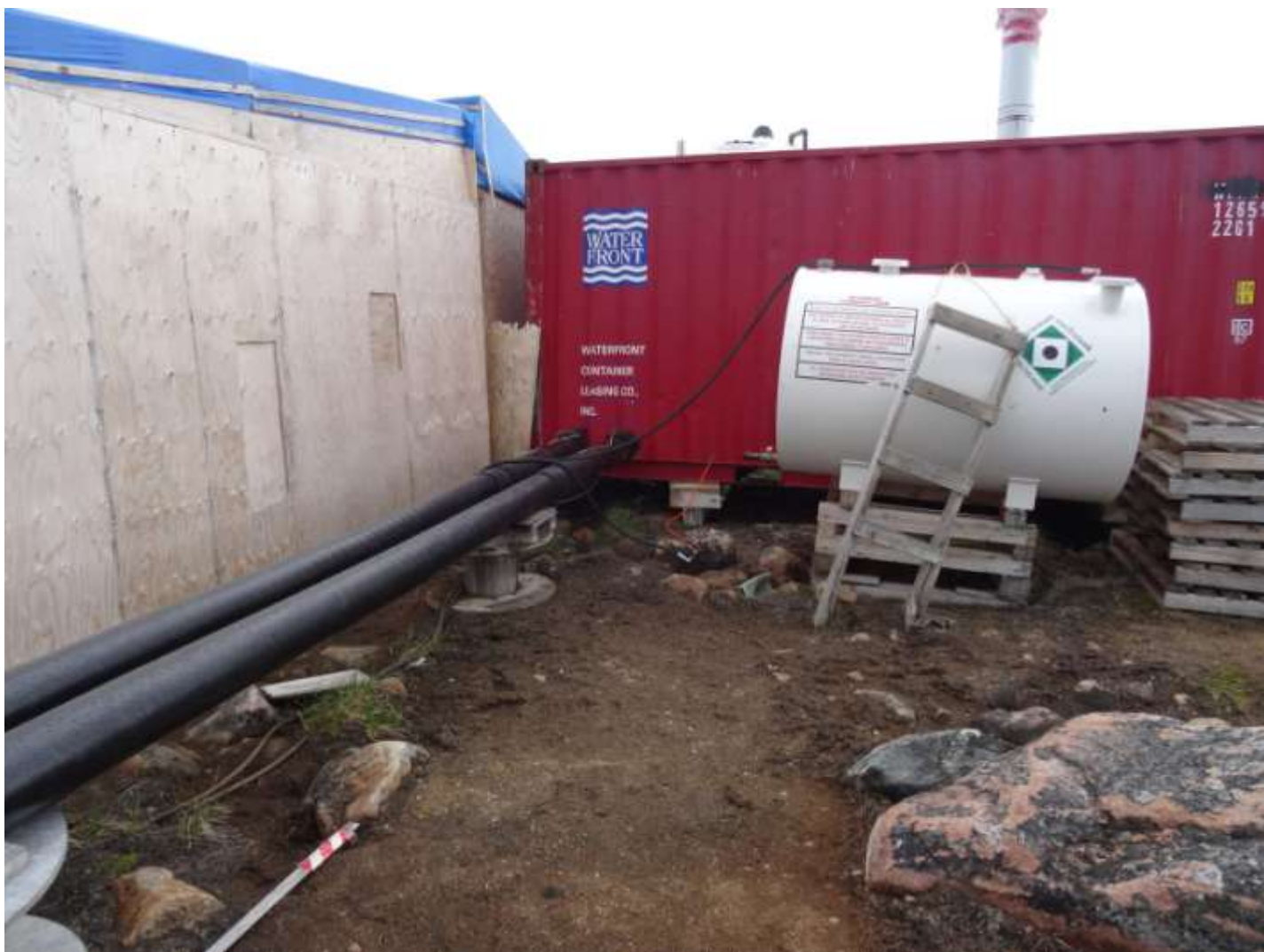
Figure 22. While tank may be double-walled, the hoses and valves are not. Secondary containment is required.
