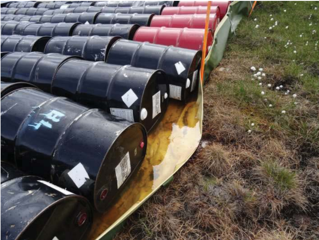
Figure 24. Collapsed side of Three Bluffs berm 2, leaking contaminated water.
