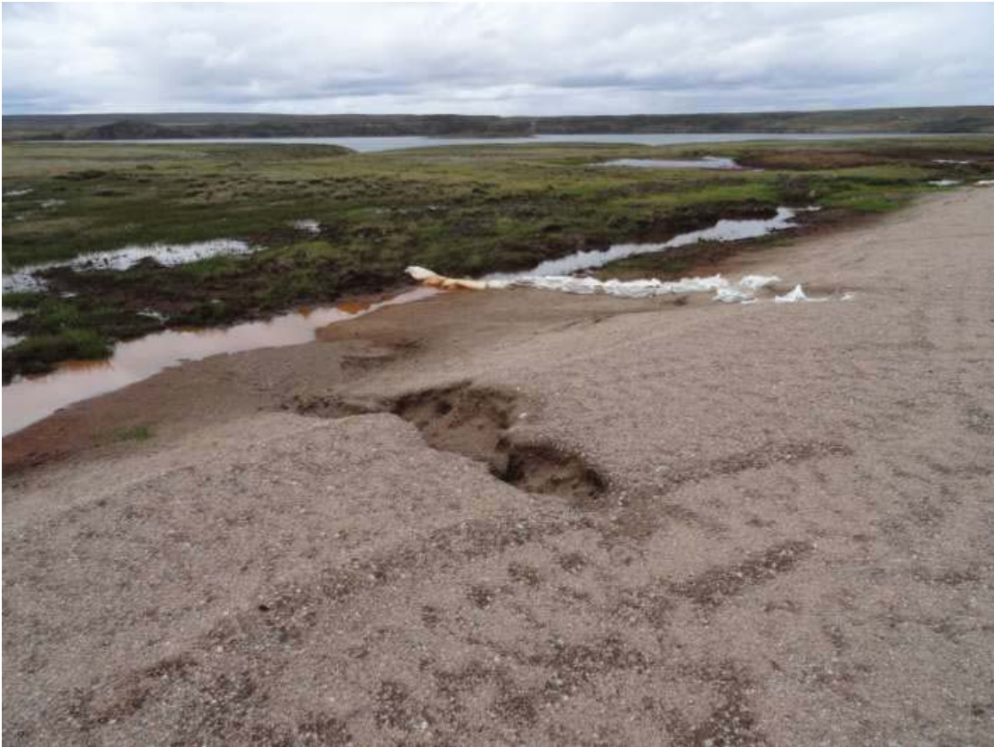
Figure 17. Permafrost degradation leading to deterioration of airstrip and sediment in the water.
