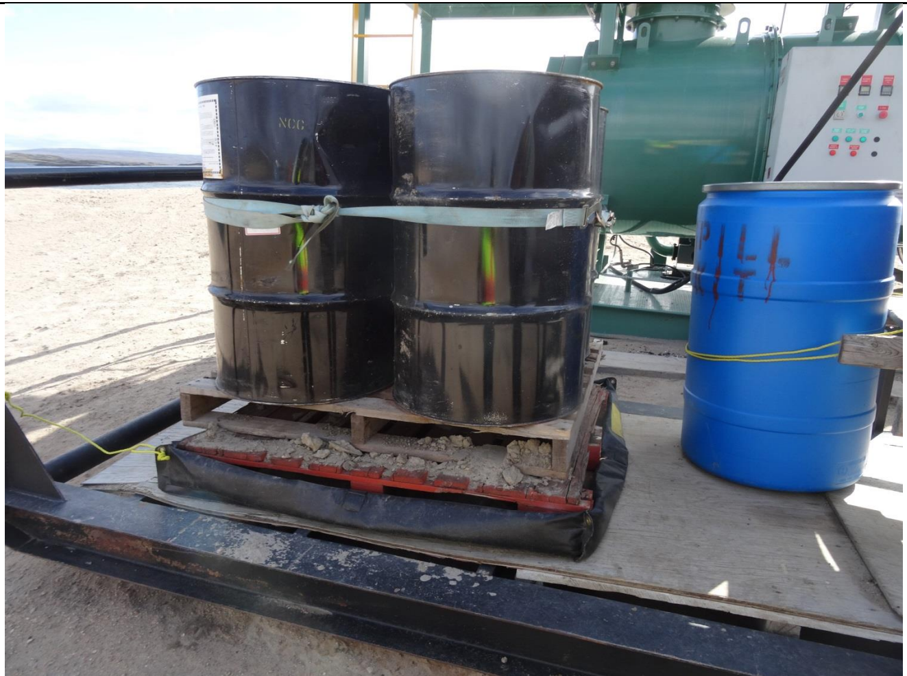
Description: Fuel Drums for Incinerator – Needs Larger Secondary Containment
