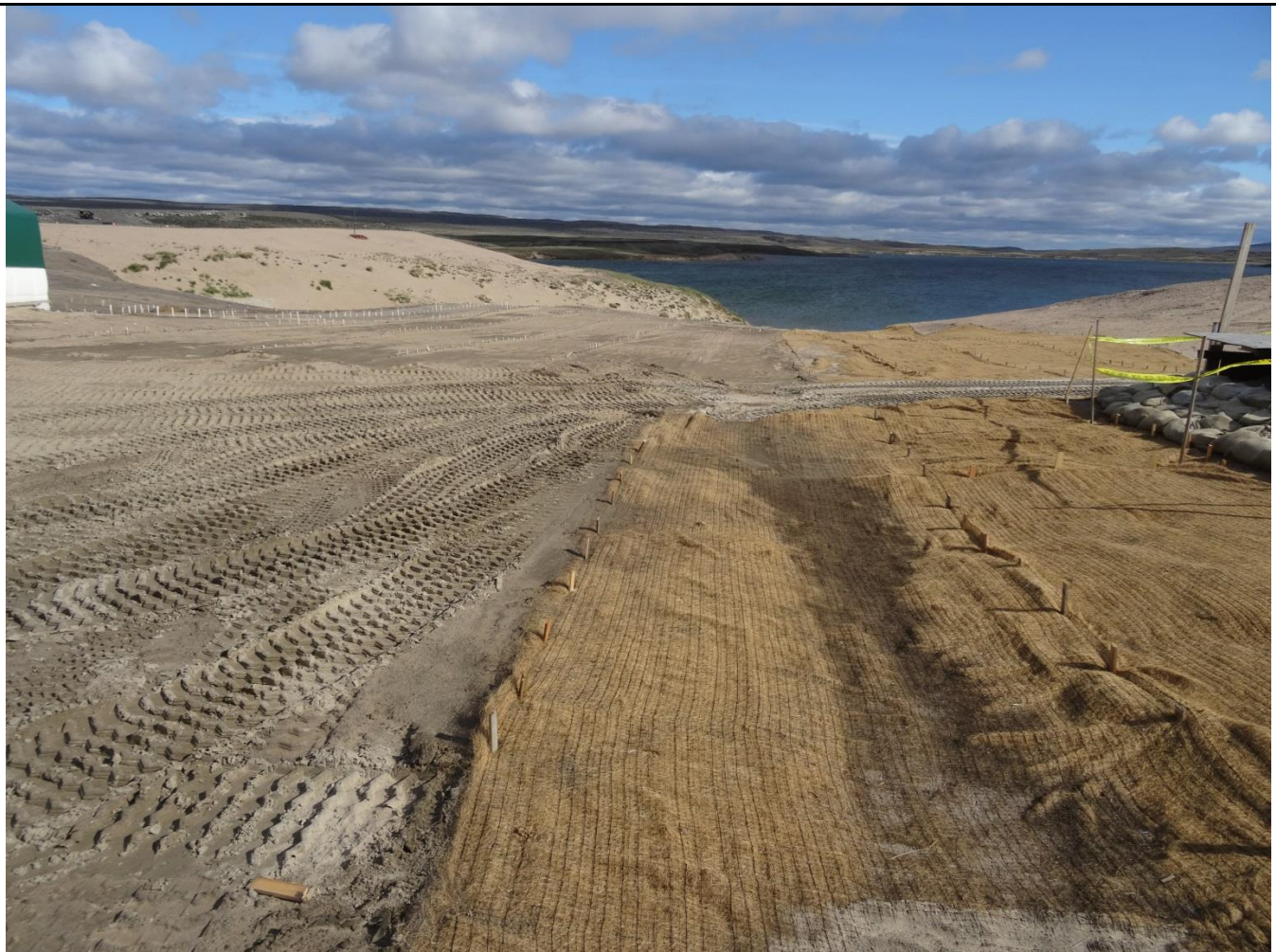
Description: Coconut Matting installed for Erosion Control as per Eva Paul’s Direction from last Inspection – also visible in Photo #2
