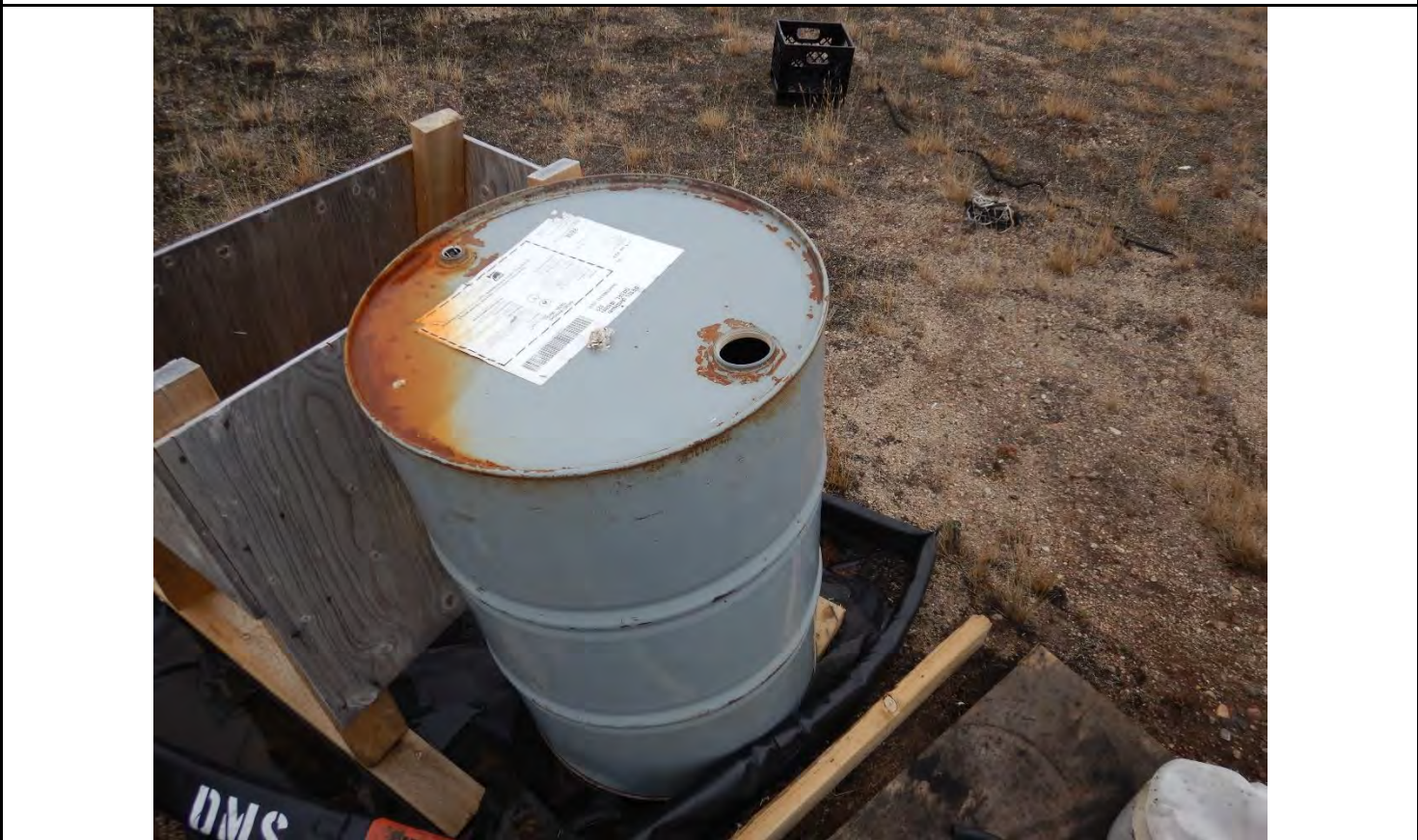
Description: wood within the containment pushing down the containment wall.
