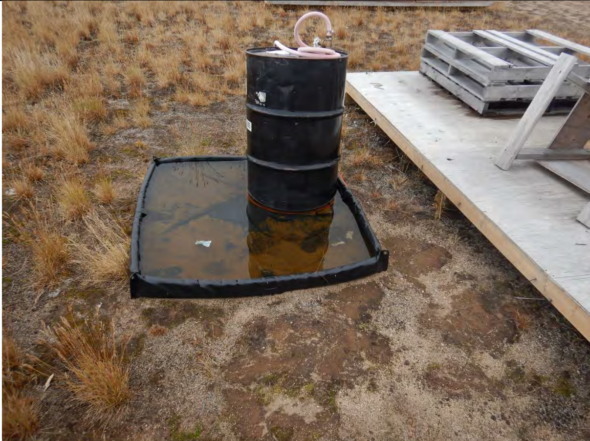
Description: secondary containment full of water.
