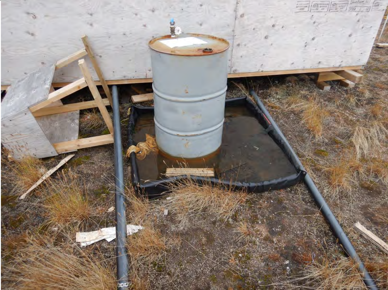
Description: secondary containment full of water.
