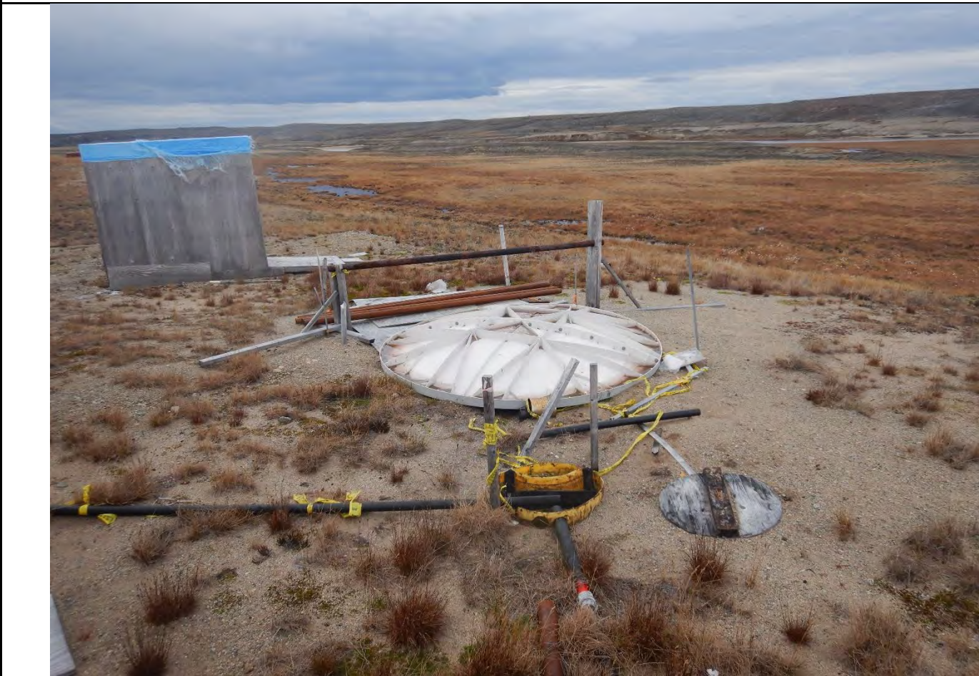
Description: sump without berms to prevent flooding.
