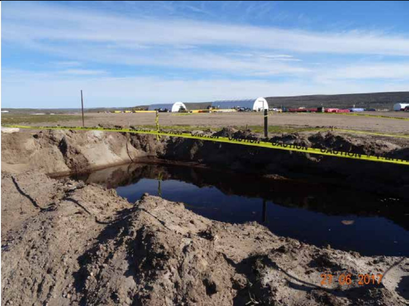
Description: Temporary sump in use for storing WWTP effluent.
