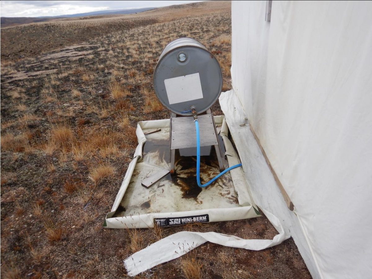
Description: heating stove tank without required covering and damaged secondary containment.
