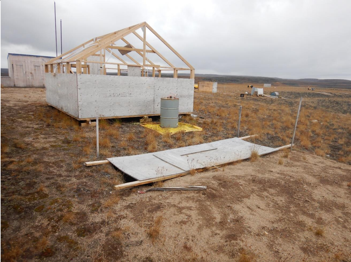
Description: partially covered sump and damaged secondary containment.
