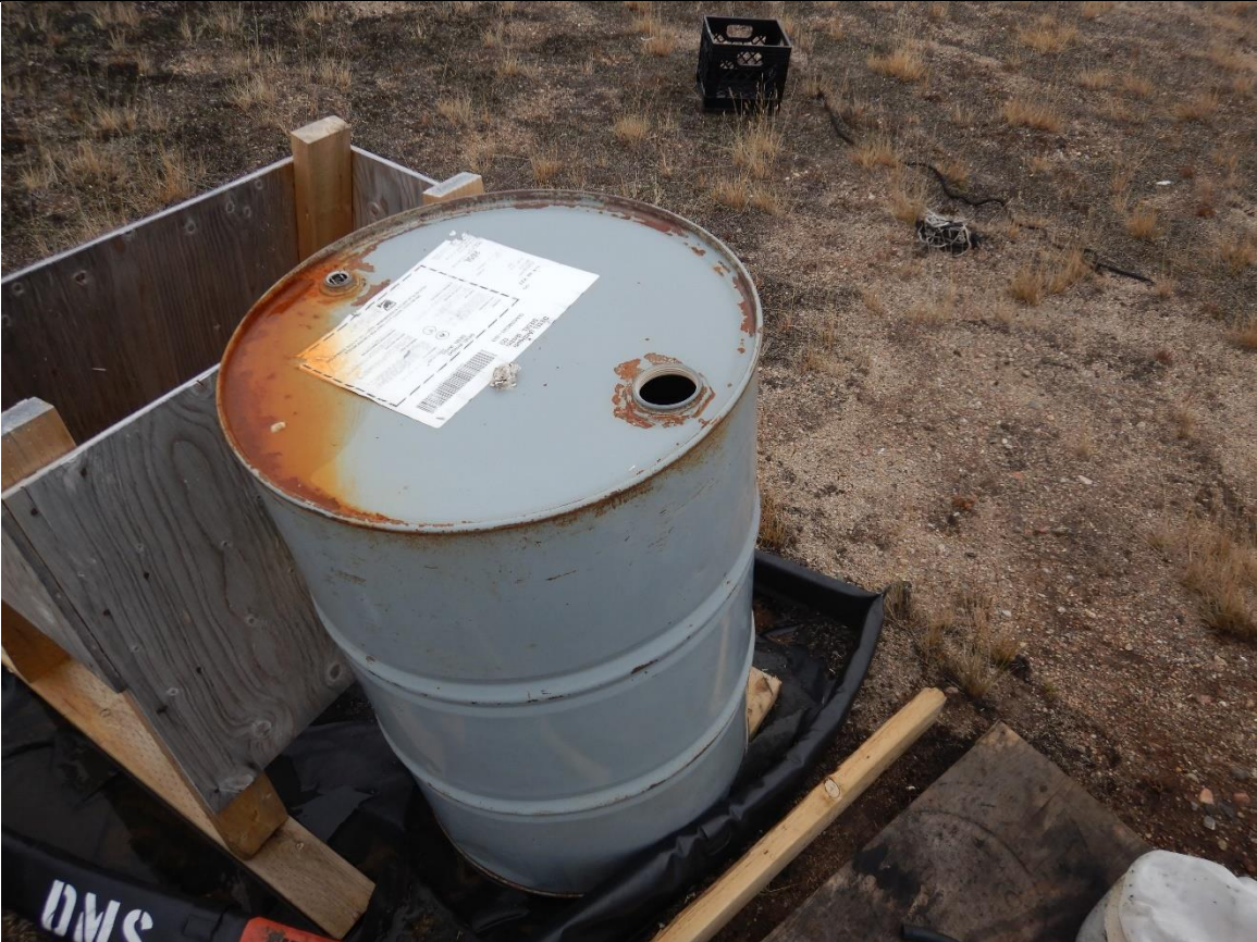
Description: wood within the containment pushing down the containment wall.
