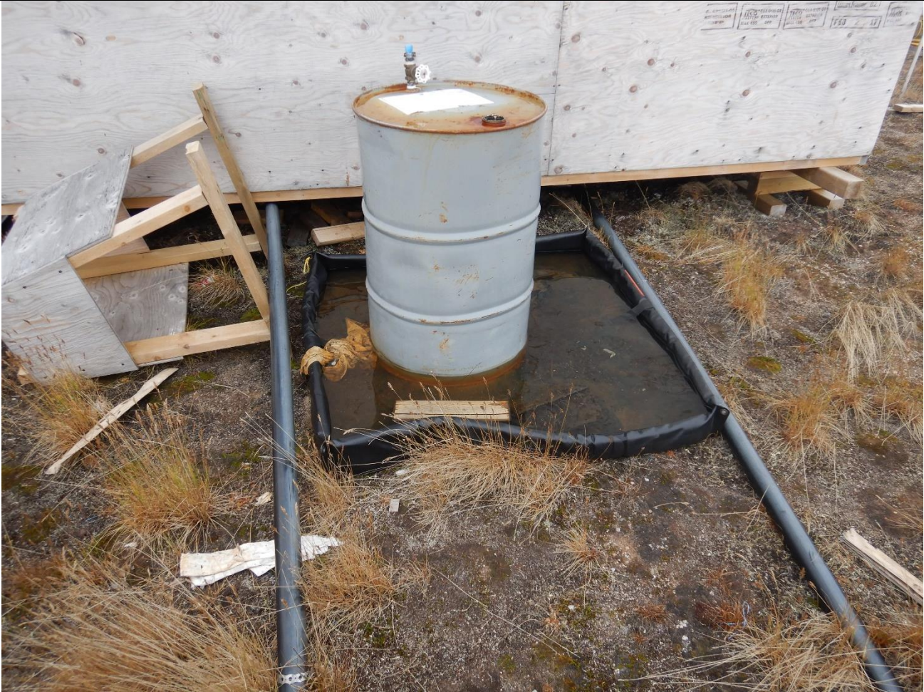
Description: secondary containment full of water.
