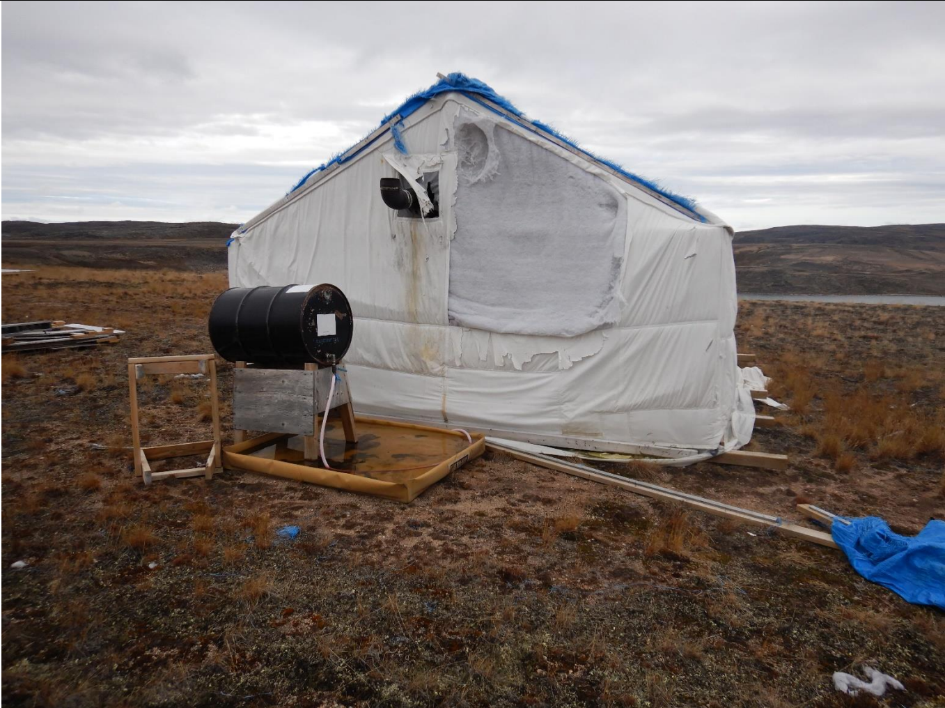
Description: heating stove tank without required covering.
