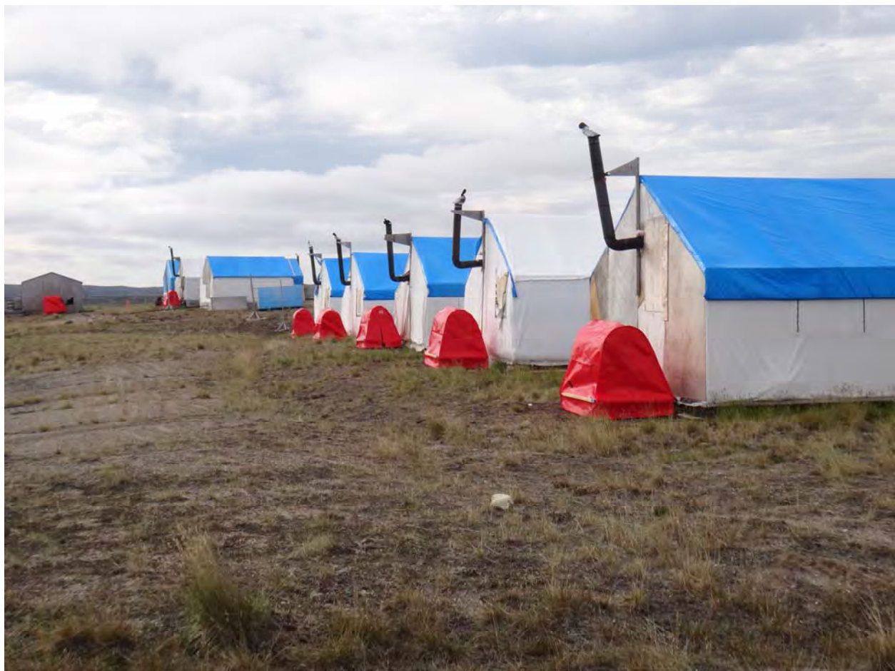
Figure 1. Secondary containment at the tents installed in 2012.
