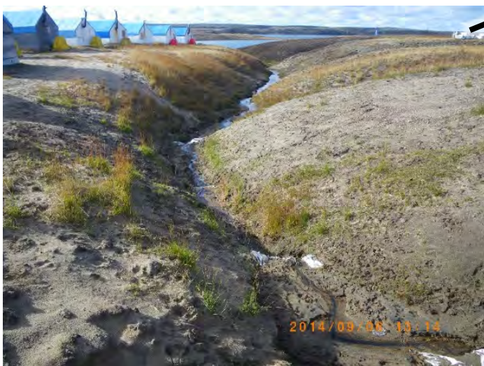
Natural gully along the east side of Hayes Camp. Surface water runoff flowing over the top of these sandbag filter dykes due to the retained sediments
