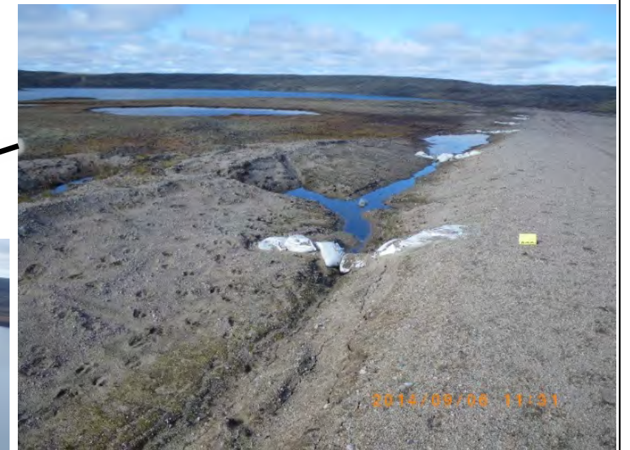
Permafrost degradation due to ponded water within the drainage ditch along the west side of the Three Bluffs Airstrip
