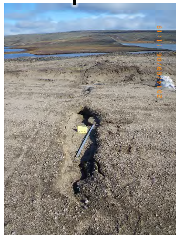
Erosion channel and piping at the crest of the runway
