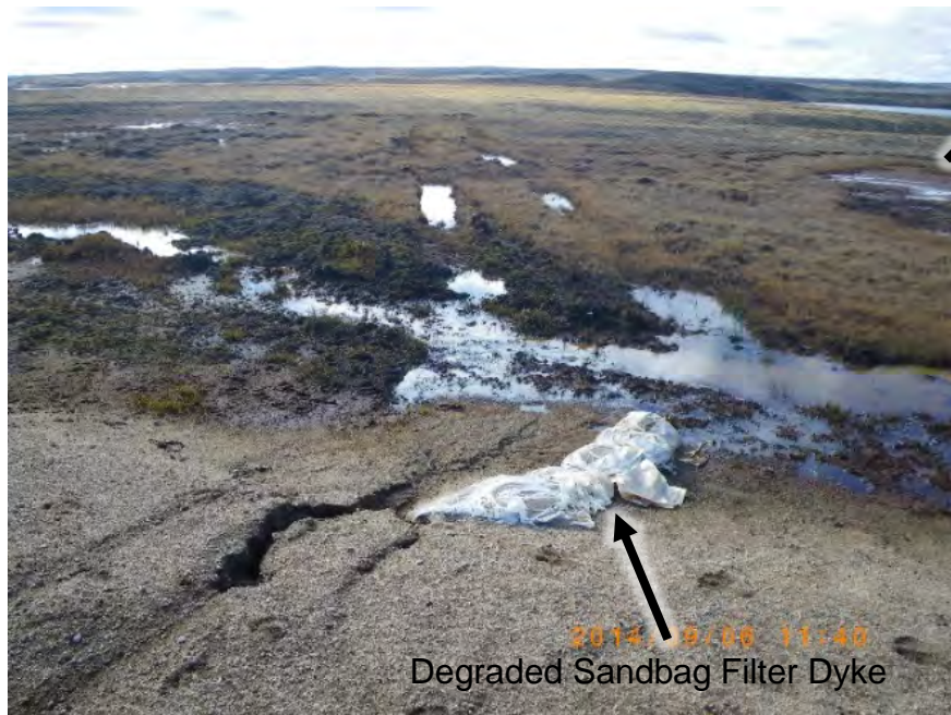
Erosion channel at the edge of the runway and permafrost degradation from a tracked vehicle in the background
