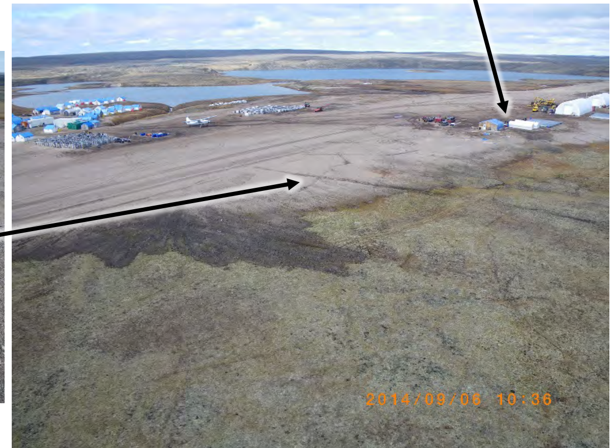
Permafrost degradation within the apron due to ponded water
