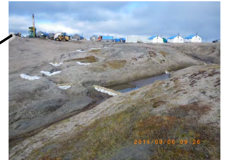
New sandbag filter dykes within the natural gullies at the south end of Hayes Camp
