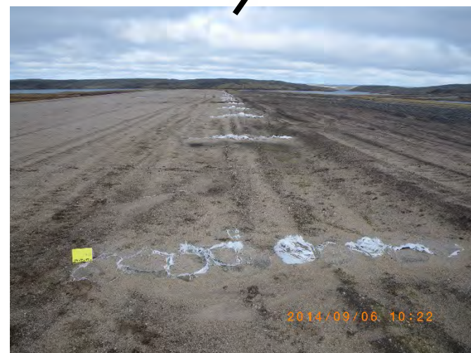
The sandbag dykes have decayed and are non-functional
