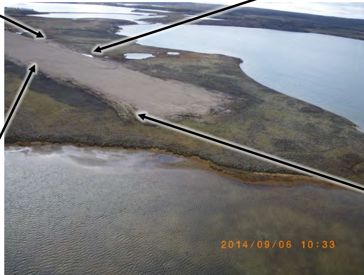
Permafrost degradation due to ponded water within the drainage ditch along the west side of the Three Bluffs Airstrip
