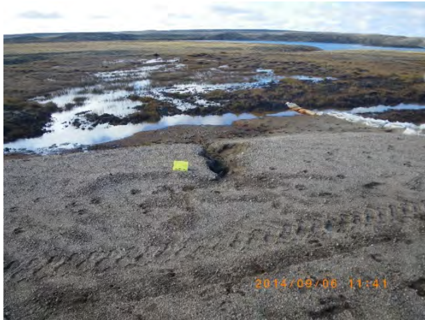
Erosion channel at the edge of the runway
