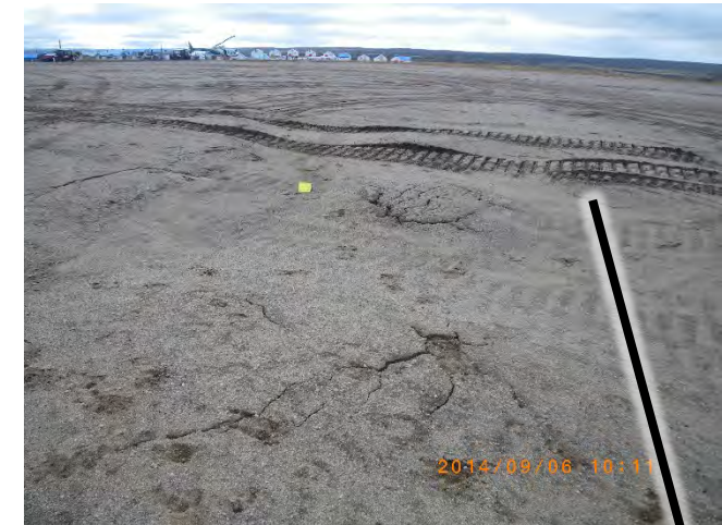
Permafrost degradation within the apron due to ponded water
