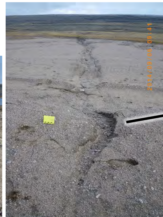
Erosion channel connected to a melted ice wedge
