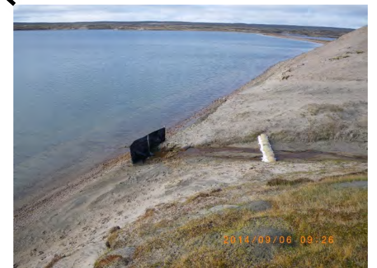
The newly installed sediment control structure at the outlet of the natural gully at the south end of Hayes Camp
