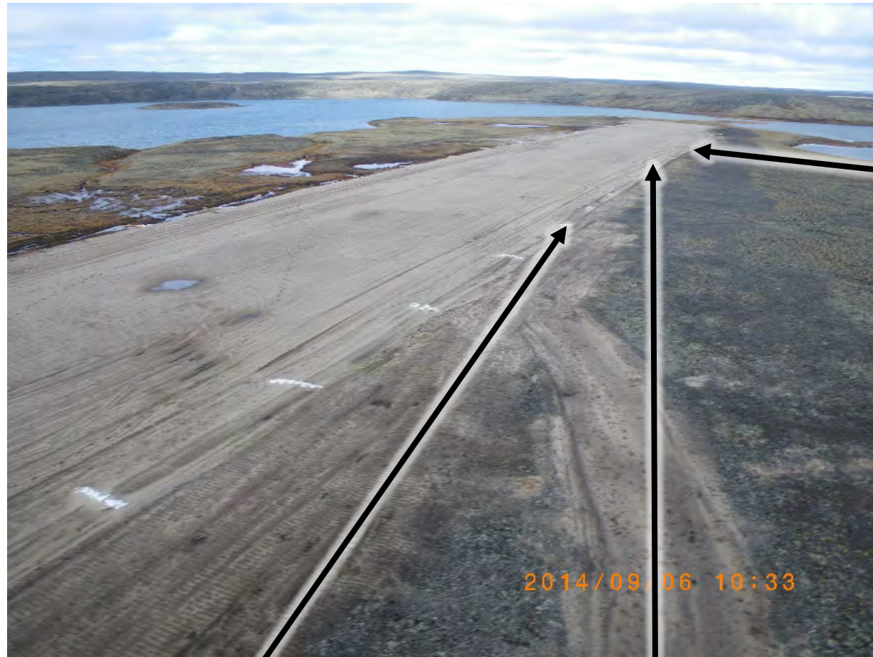
No further melting of the ice wedge suggests steady state conditions have developed
