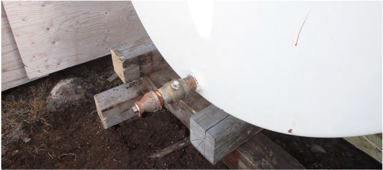
Figure 29 – Fuel hoses were removed from the base of the tank, the valve handle removed and a bung installed to prevent any accidental discharge.
