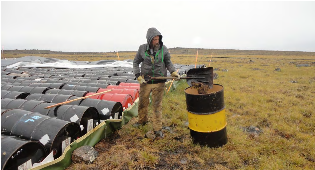
Figure 25 – Contaminated soil being removed from hydrocarbon spill which occurred as a result of Berm 2 overflowing.
