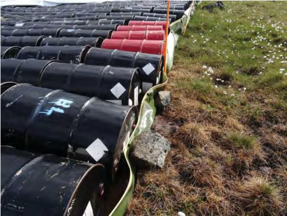
Figure 25. I propped up the side for a temporary fix. More precipitation will cause further overflow of contaminated water.
