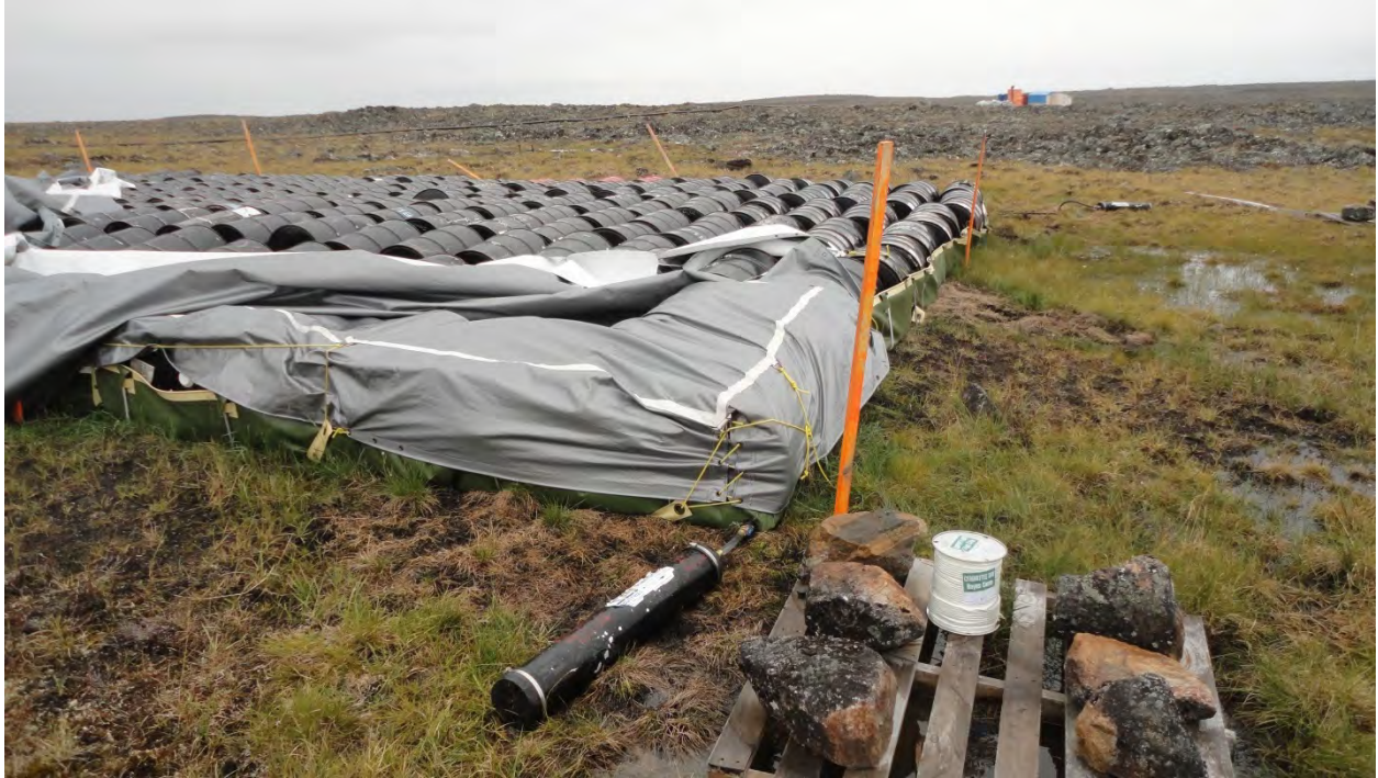
Figure 18 – Two 'Rain Drain' filters attached to Berm 2 (2014 Inspection Report Figure 24) to treat hydrocarbon contaminated water
