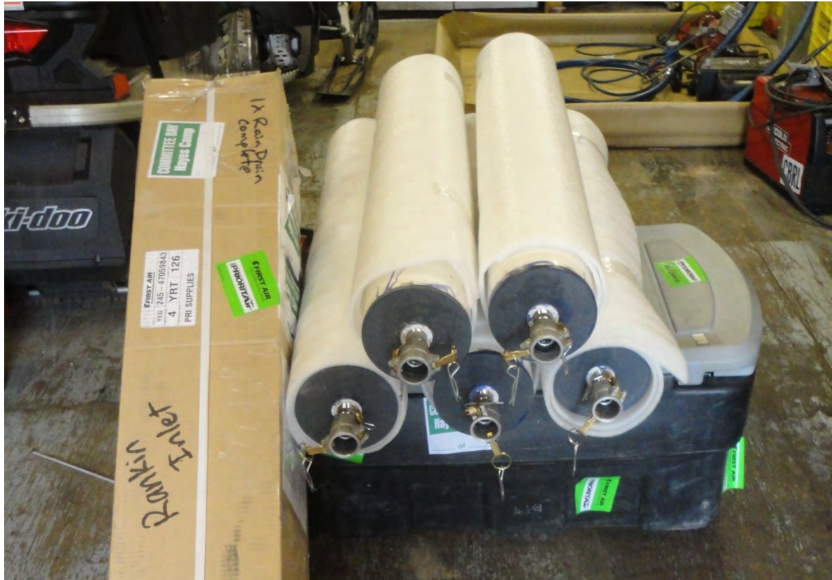
Figure 4 – New rain drain filters ready for installation
