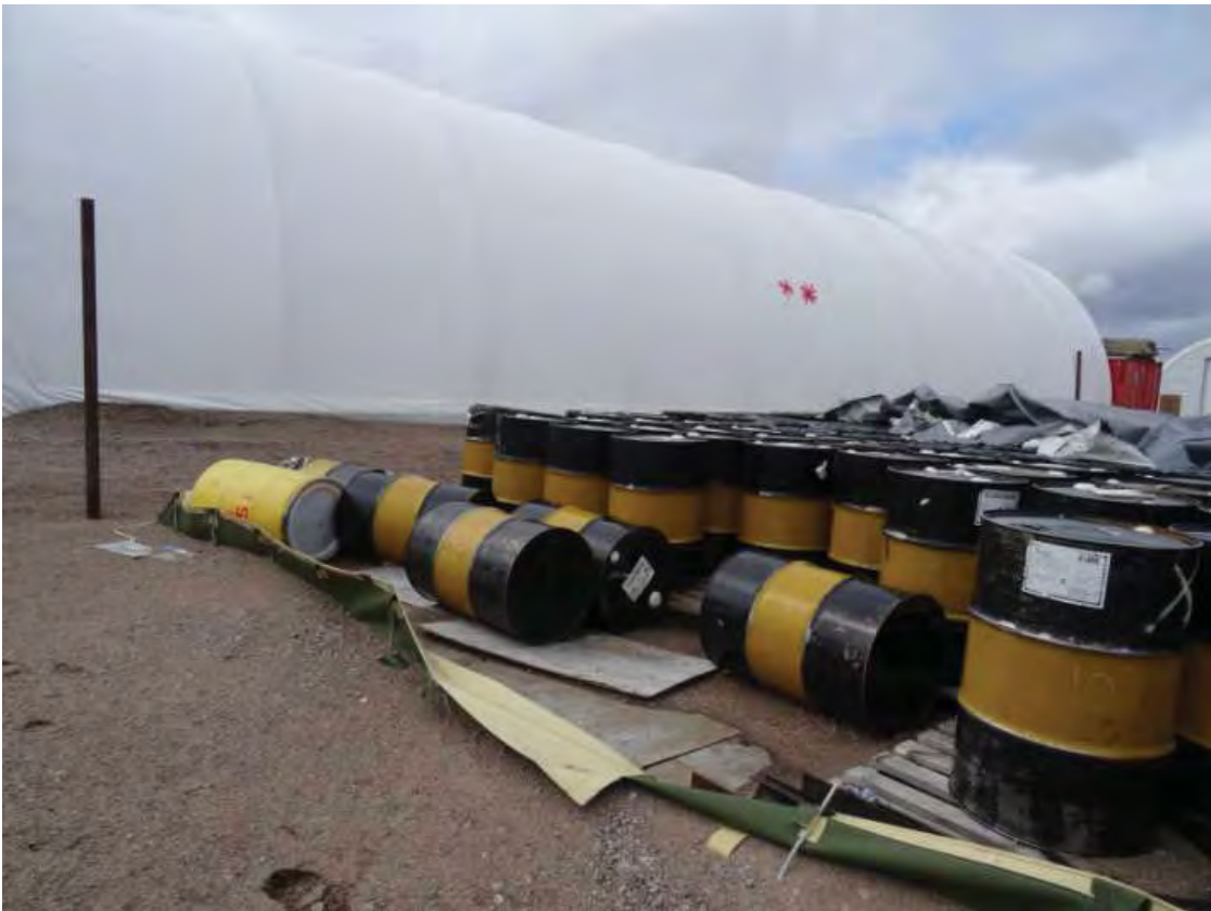
Figure 10. Hayes berm collapsed.
