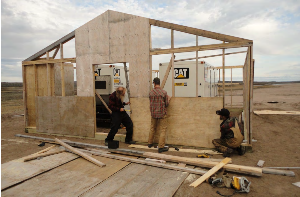
Figure 13 – NCGC staff rebuilding Generator shack. Generators repositioned enable more suitable and wind resistant construction.
