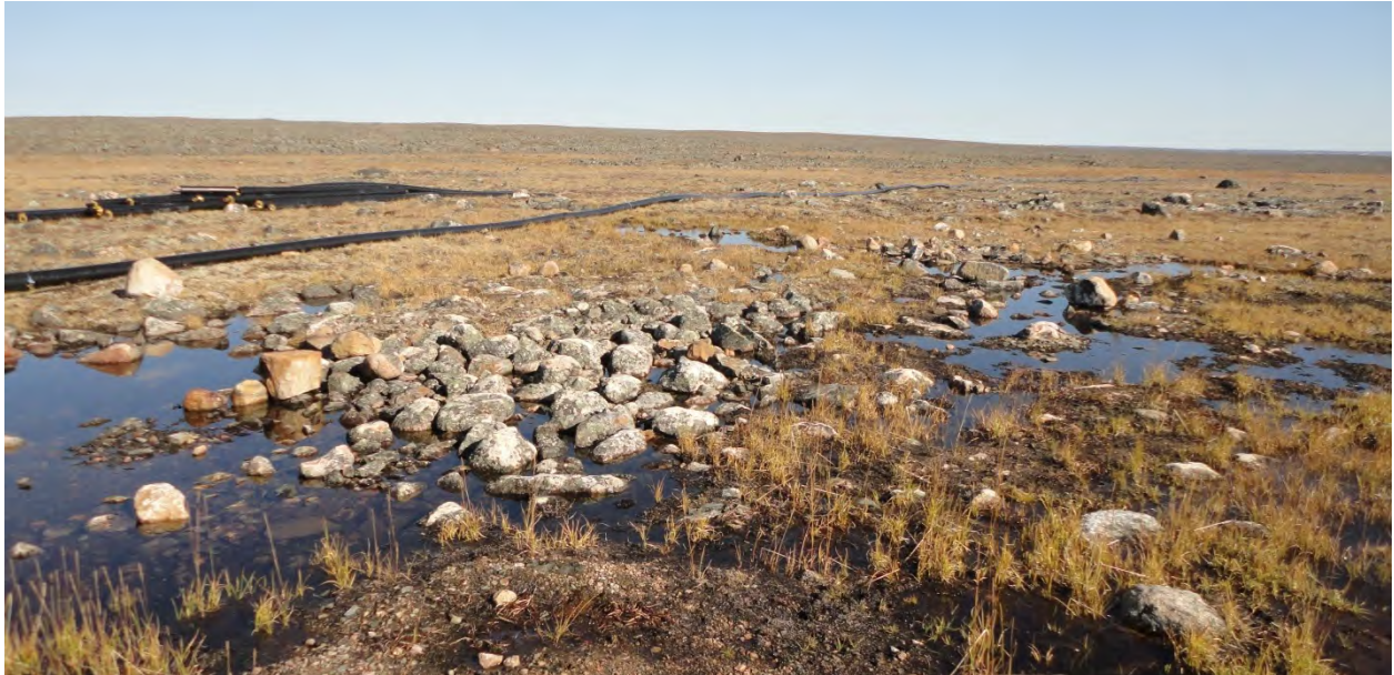
Figure 27 – Site of 2012 hydrocarbon spill. Absorbent matting was removed. Holes were backfilled to best extent possible within the natural wetland area (See 2014 Inspection Report Figure 28).
