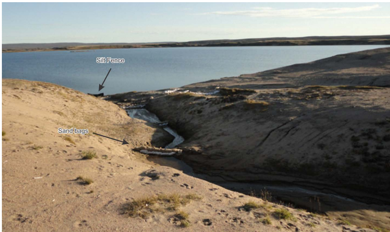
Figure 10 – Erosion control measures implemented (view southwest)
