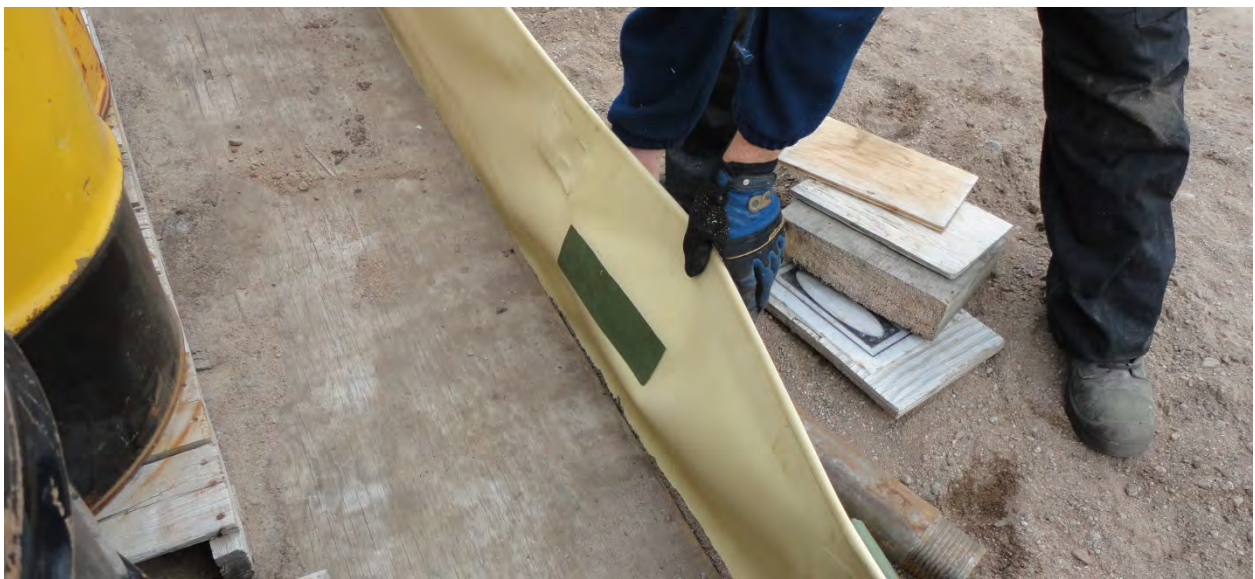
Figure 7 – Patching damaged fuel berm
