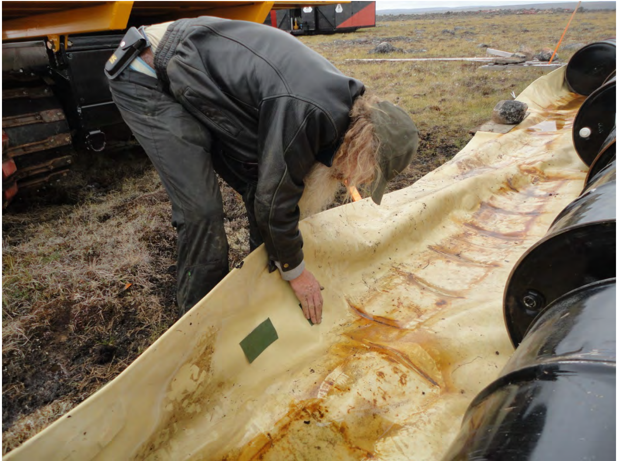
Figure 19 – Repairing damaged fuel berm
