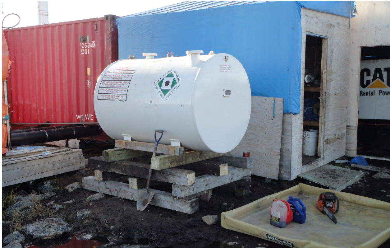
Figure 28 – Double walled fuel tank at the boiler repositioned on a solid base
