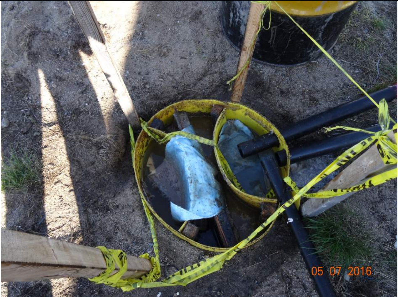
Description: Grease trap at Bullion Camp shows signs of overflowing.
