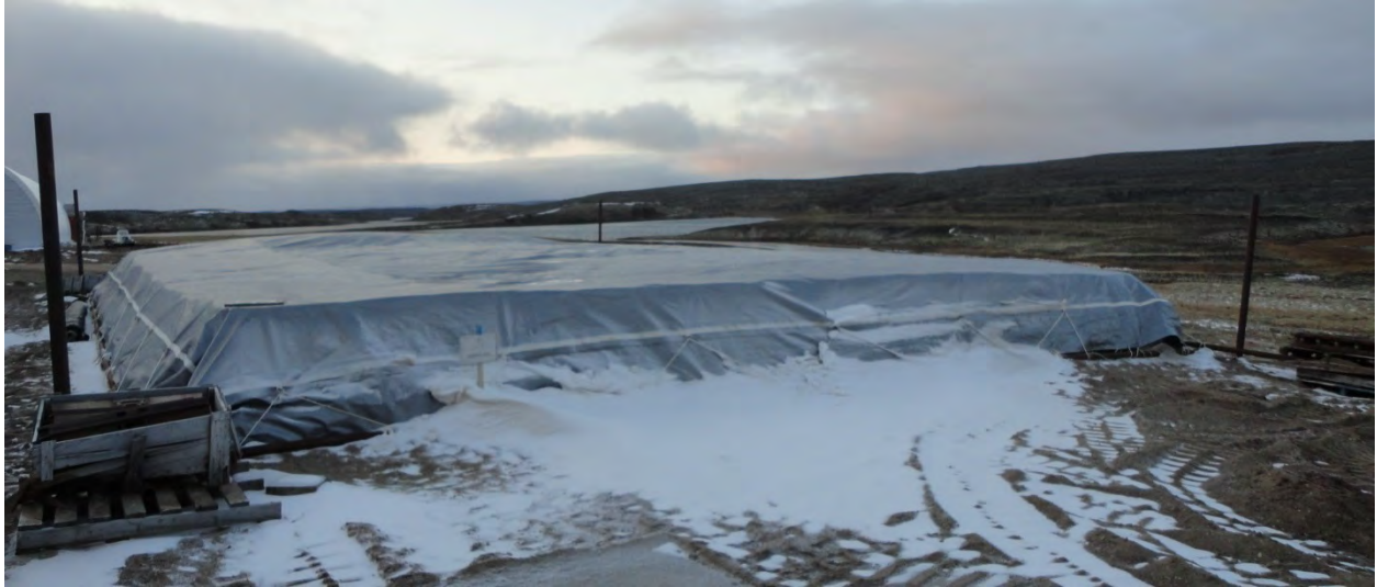
Figure 8 - Waste Oil / Fuel Berm on eastern side of Quonset 1 (Hayes Camp) with cover repaired and reinstalled. This is fuel berm shown in 2014 Inspection report Figure 10. Drill steel and scrap metal Caterpillar track pads have been used to provide additional anchor points to hold cover on in high winds.
