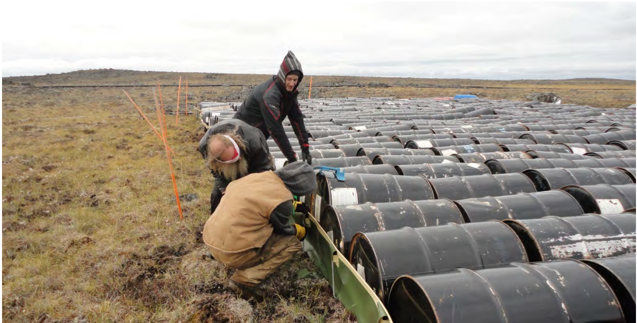
Figure 20 – Replacing damaged support brackets on berm 3 at Three Bluffs.
