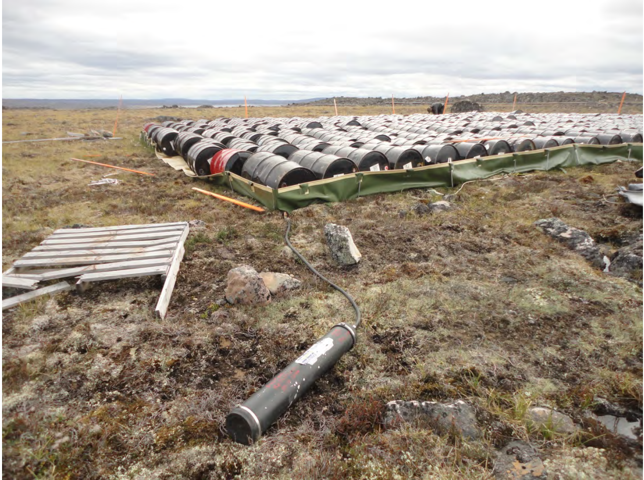
Figure 21 – Fuel berm 3 at Three Bluffs. The row of fuel drums on the far left was repositioned and additional wall support brackets added to ensure berm stability.
